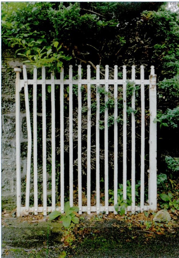
North half of front gate. One of a pair of fine wrought iron gates
