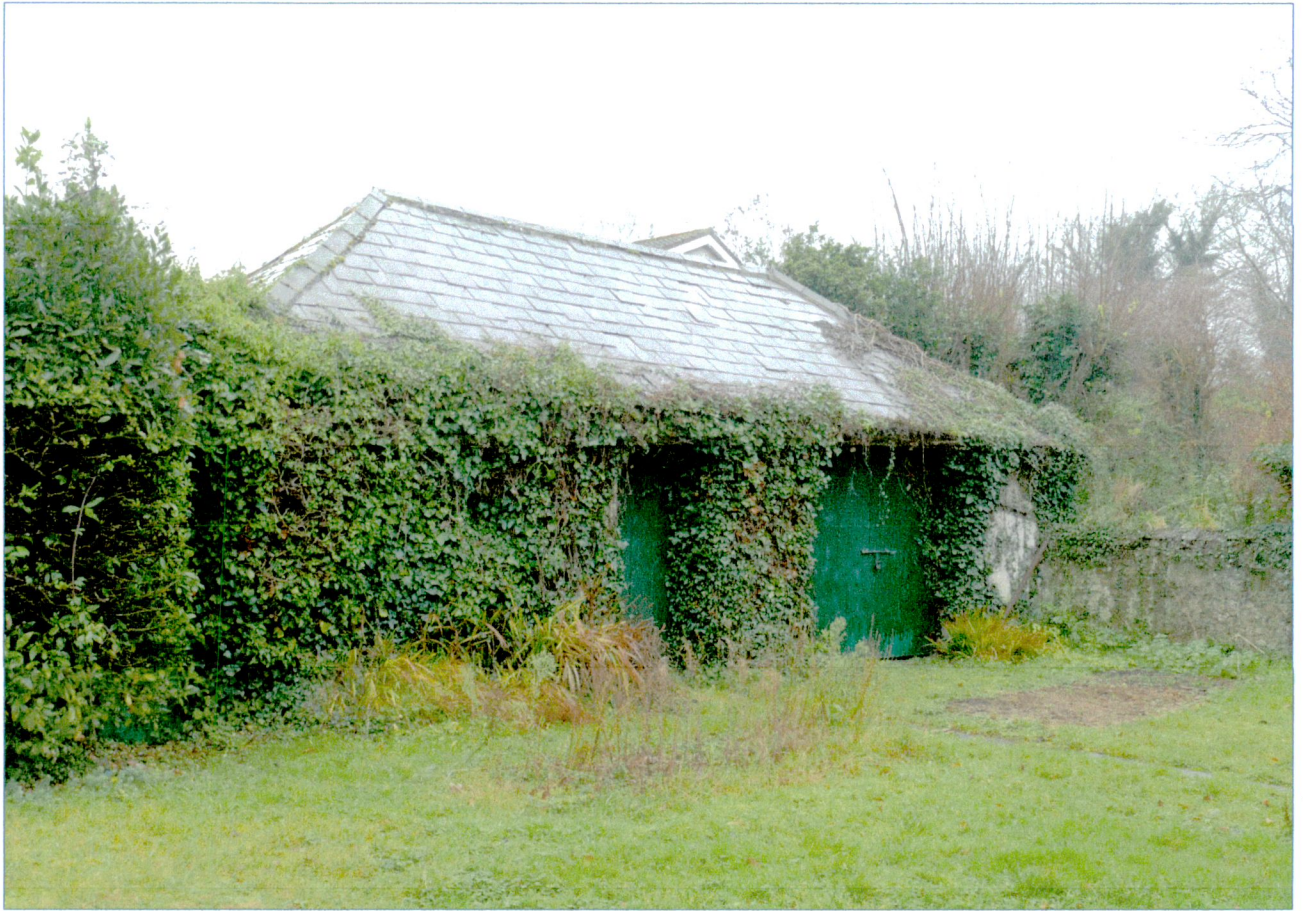
South west outbuilding. It is proposed to overhaul and repair this outbuilding.
