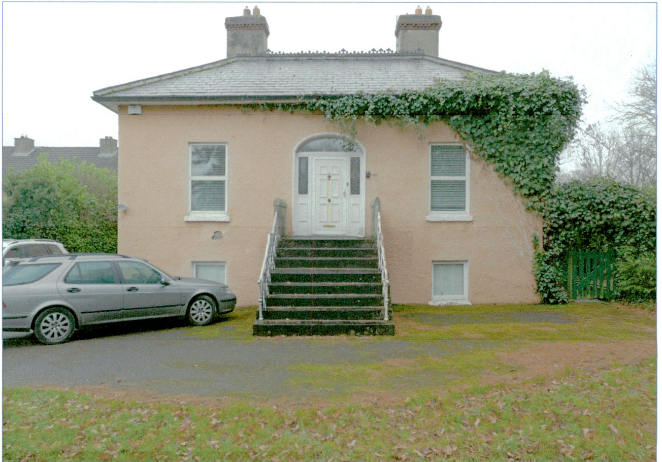
Front (west) facade. It is proposed to replace the existing uPVC windows with timber l-over-l up-and-down sash windows detailed appropriately and to replace the modern door and doorcase with a timber door and doorcase of a design and detail appropriate to the period of the house
