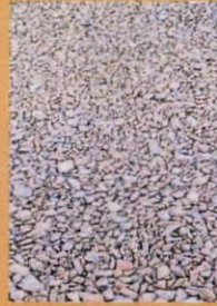
Laying course 2-6mm clean crushed stone
