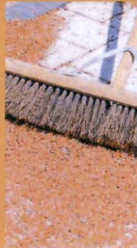
Surface Dressing 2-4mm clean crushed stone
