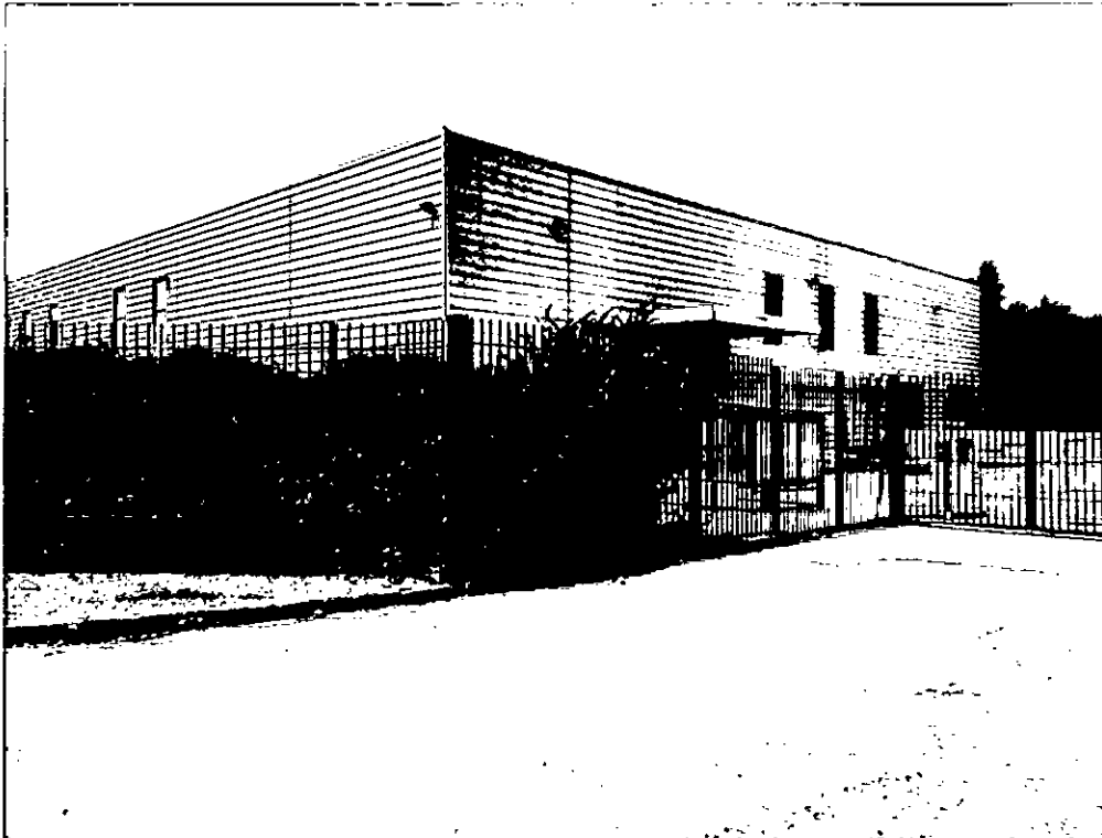
Photo 1. Existing building on site.
