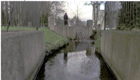
Plate B15 A significant instream barrier present on Section 007 on the River Poddle at Kimmage Manor
