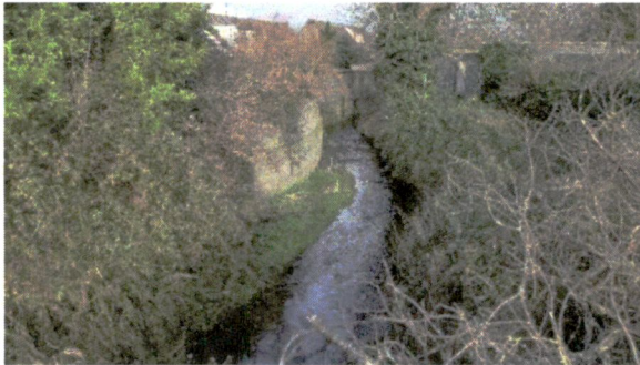
Plate B13 Section 005 on the River Poddle was historically straightened & deepened (no otter signs recorded)
