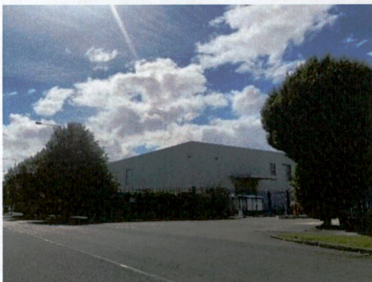
Plate 1 - Entrance from internal estate road
