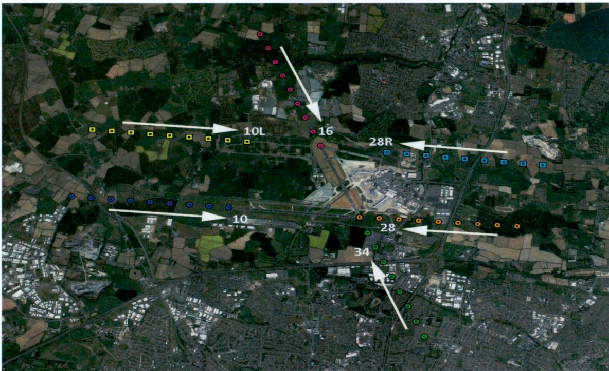
Figure 6: Aerial view (Google Earth Pro) showing 2 mile approach lines to runways at Dublin Airport (at ¼ mile intervals) as assessed by SGHAT. Includes the proposed northern runways 10L and 28R.
