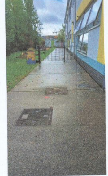
6 EXISTING GARDEN LOOKING SOUTH Scale NTS
