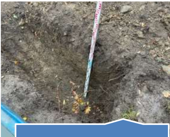
BRE test hole
