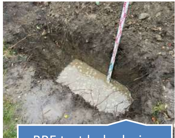
BRE test hole during testing
