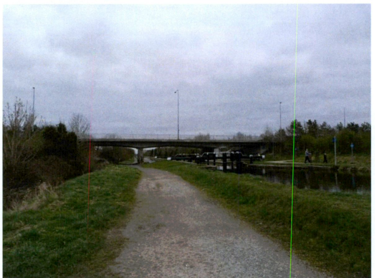
Plate 24. The Grand Canal, view to east, with bridge of R113 in background.
