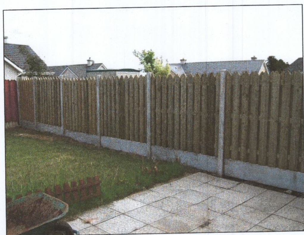
1800mm high vertical timber fencing panels with concrete plinth and post
