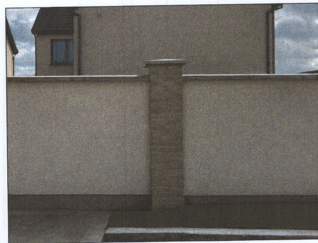
1800mm high rendered wall with brick capping
