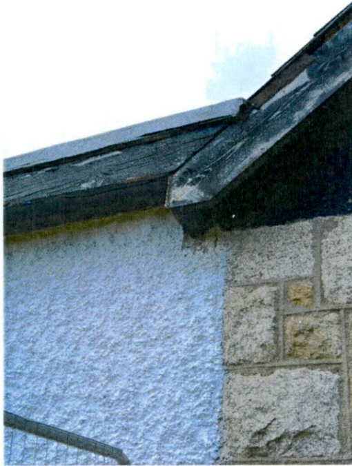
existing cottage and existing rear extension
