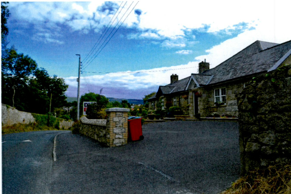
-Street Elevation, Whitechurch Road
