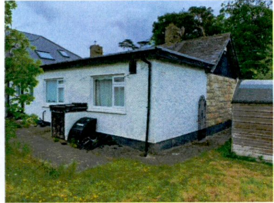
-Rear Elevation, No.626 Whitechurch Road
