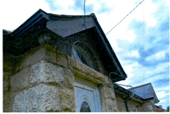
-Rear Elevation, No.626 Whitechurch Road
