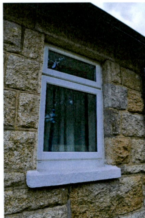
-Example of UPVC window to be replaced
