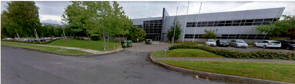
Figure 3: front (west) elevation view of the site
