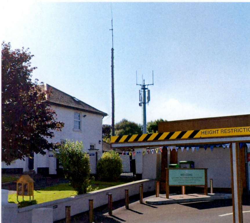
Figure1. Existing Structure in Rathcoole
