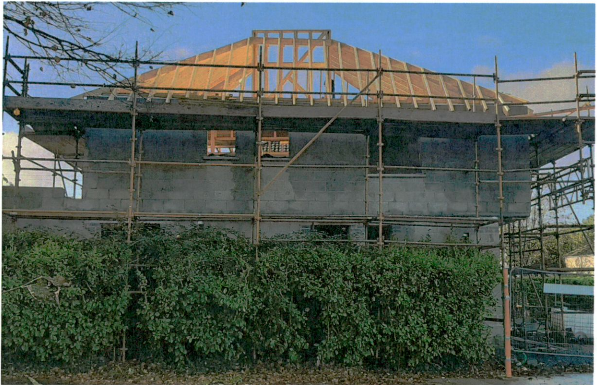
New house under construction, November 2022
