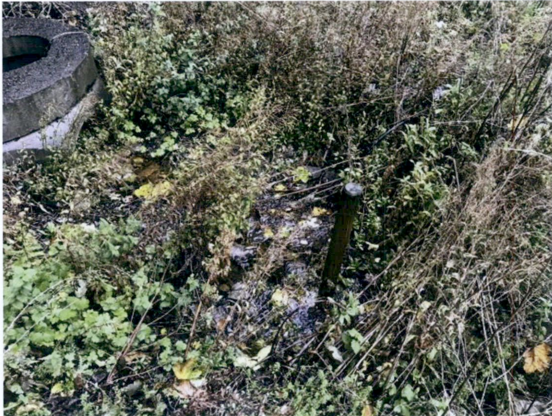
Figure 5: Open spring with concrete ring and culvert to left of image
