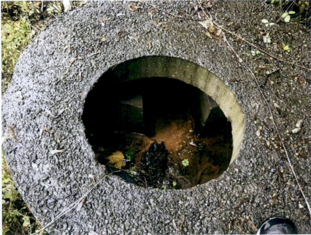
Figure 6: Concrete ring and culvert
