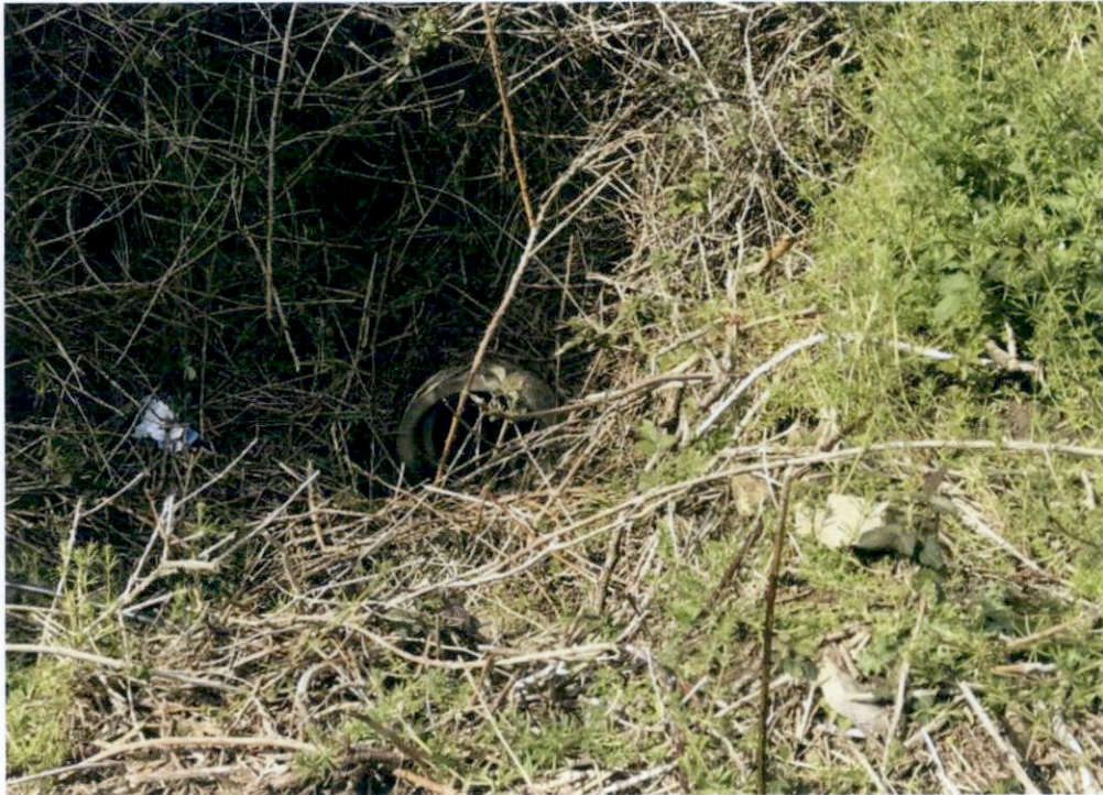
Figure 5: Pipe at northern end of ditch
