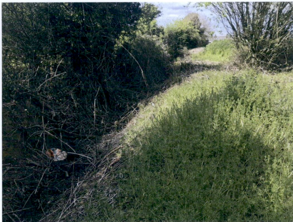
Figure 6: Drainage ditch, photograph taken 03/05/2022
