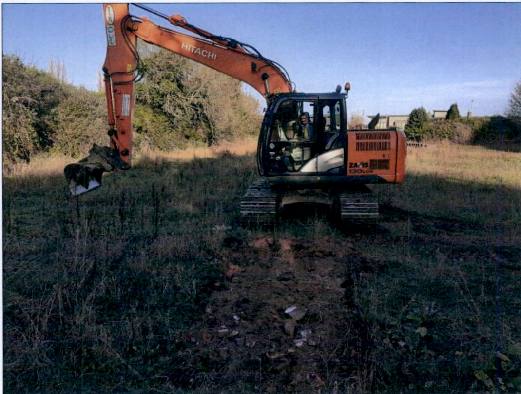
Plate 27: Trench 6 (T6) showing make-up of overburden, facing north
