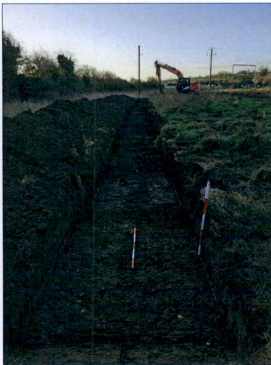
Plate 20: Trench 4 (T4), facing south
