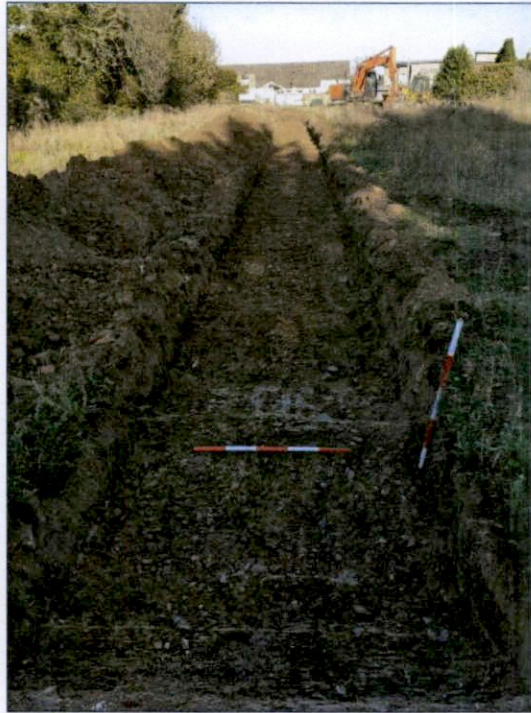
Plate 29: Trench 6 (T6) north
