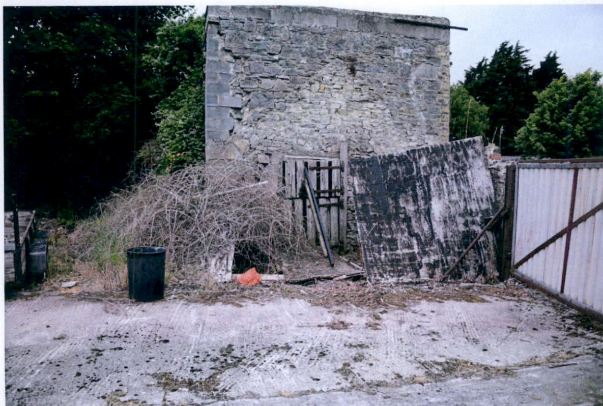
Plate 2. Buildings on site.
