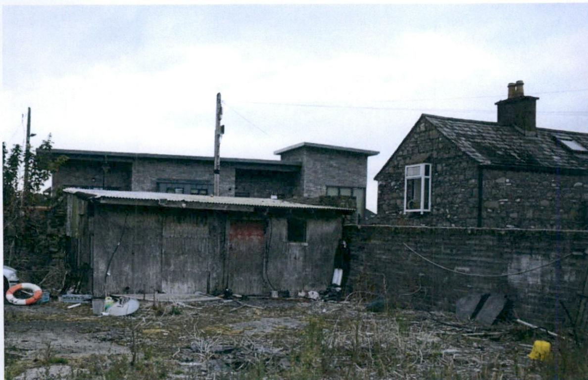
Plate 1. Buildings on site.
