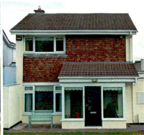
No.s 69 Monastery Drive
