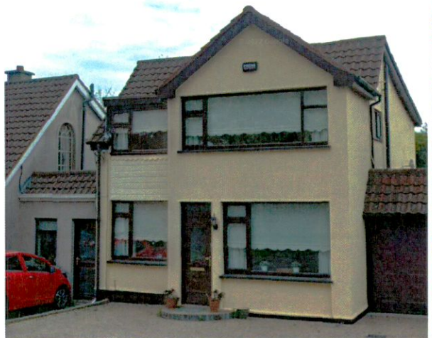
No. 62 Monastery Drive
