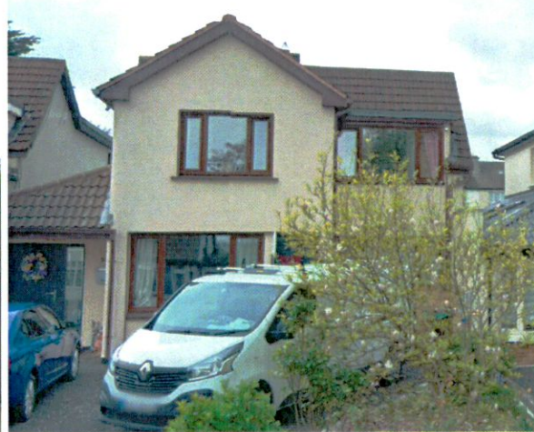
No. 29 Monastery Drive
