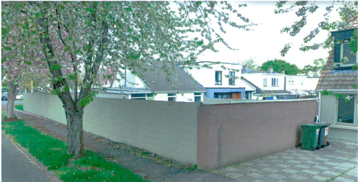
Streetview of No. 64 from the Rear
