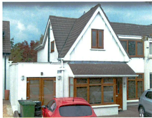
No. 77 Monastery Drive
