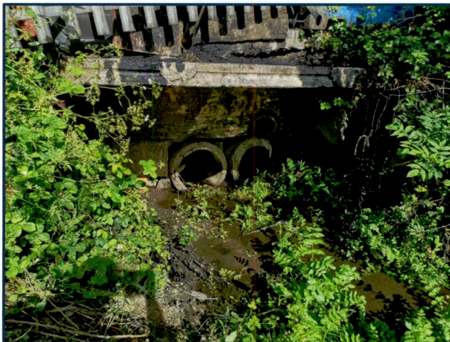
Figure 5-8 Inlet to twin-pipe culvert
