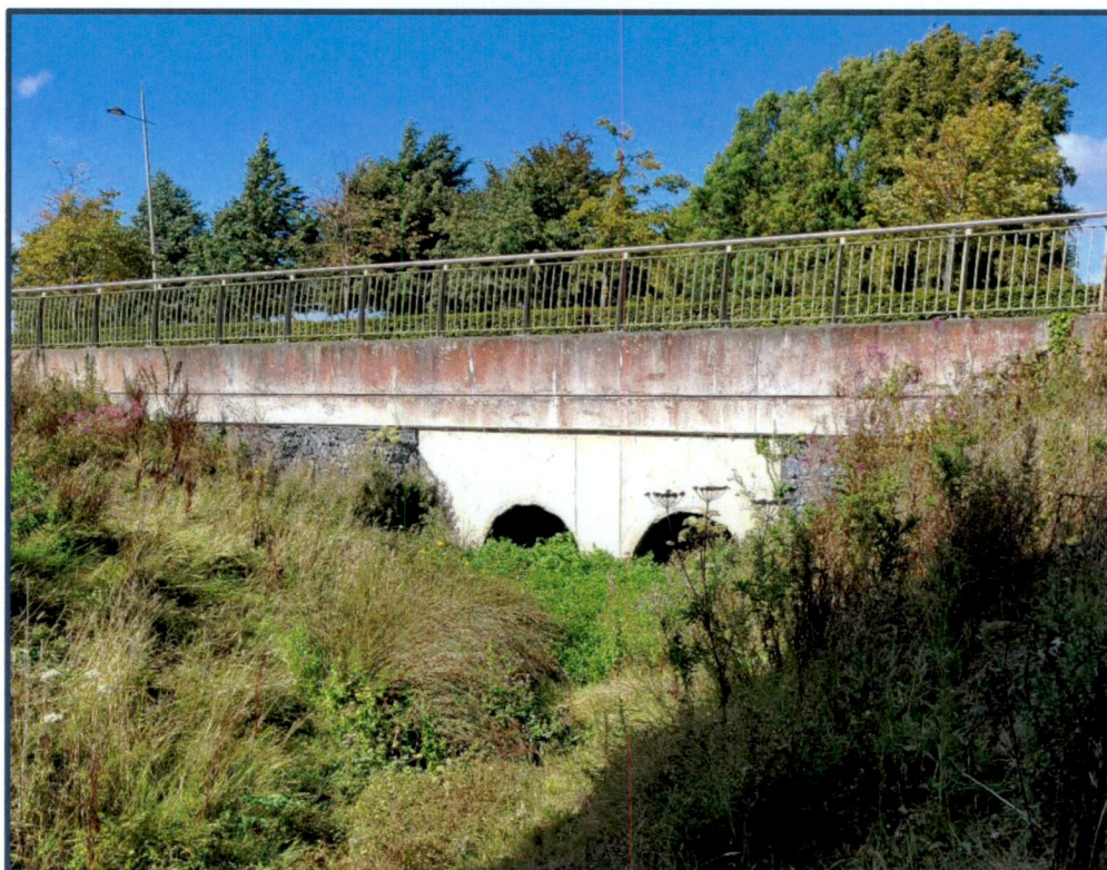
Figure 5-7 Upstream View of Culvert under Falcon Avenue
