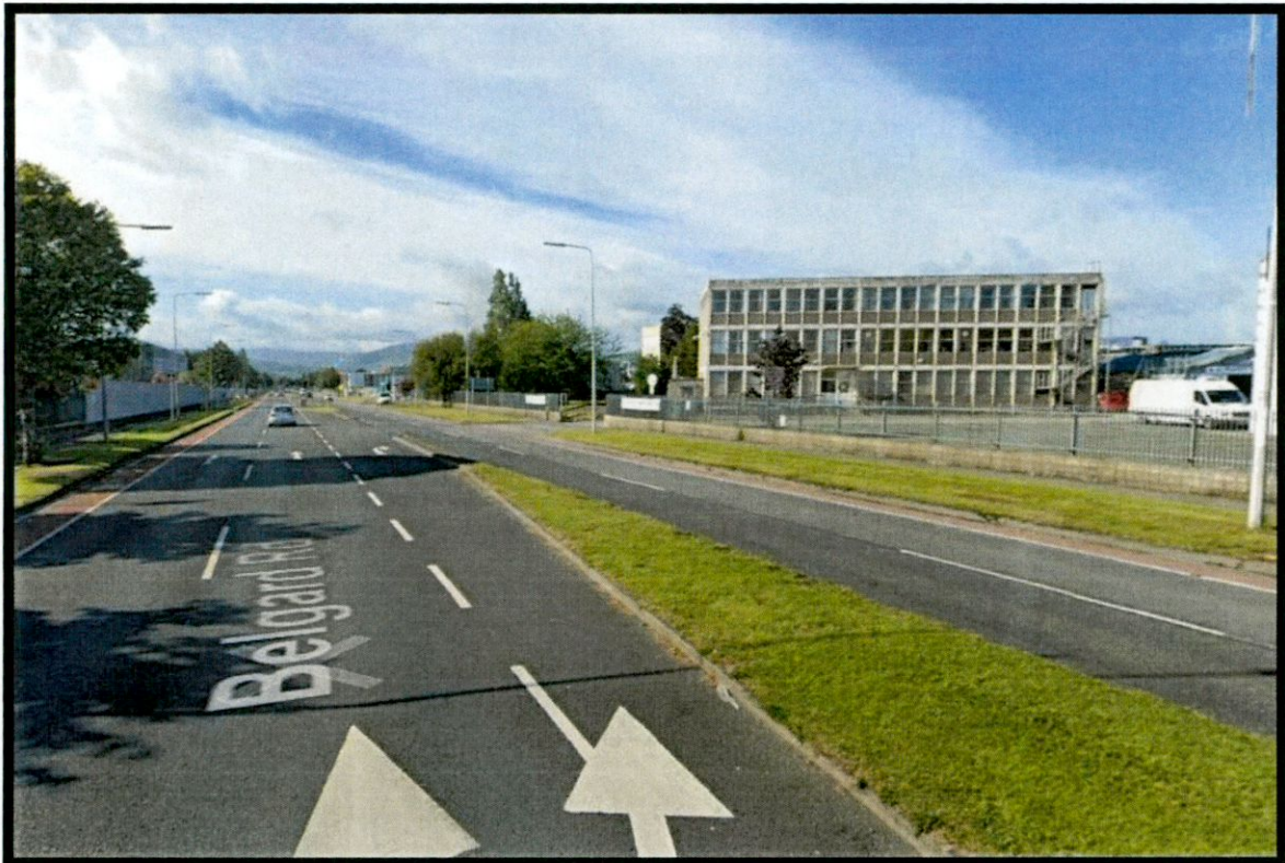
Figure 2.3 – Belgard Rd, View South, with Site on RHS
