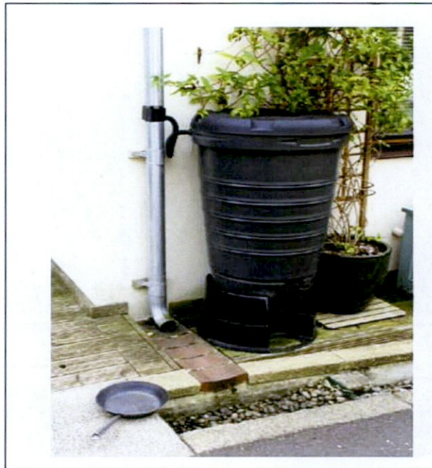
Figure 8– Rain Water Butt Detail
