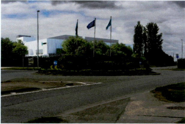
Figure 8-10: Operation Stage Year 5: Viewpoint 7 - R134 New Nangor Road at the entrance to Profile Park looking south west.
