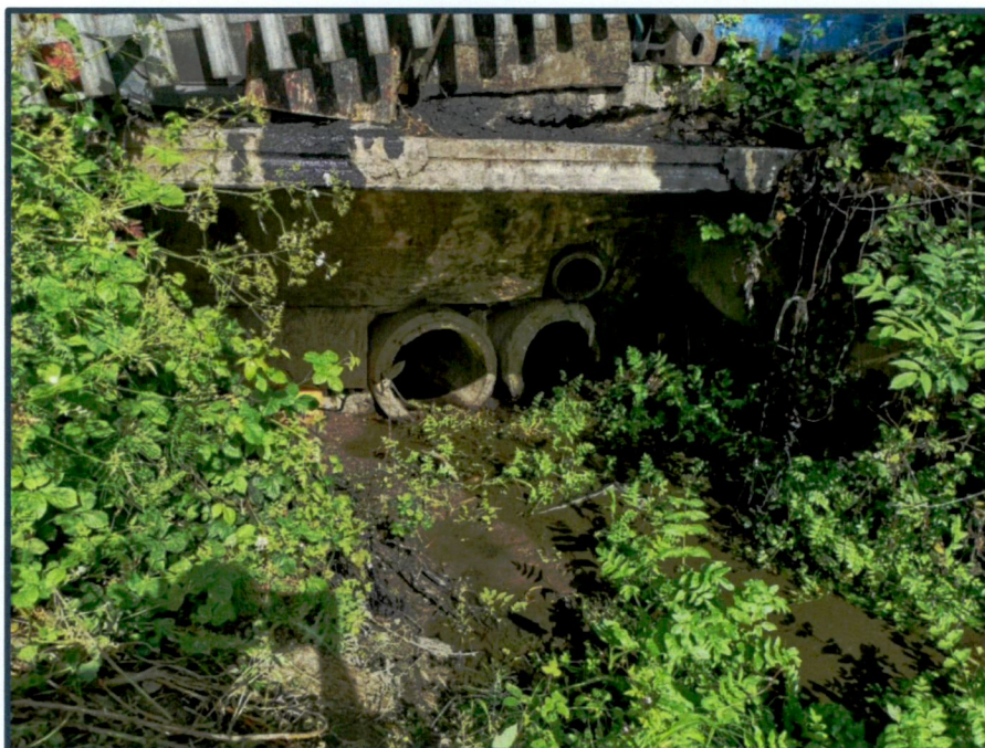
Figure 5-8 Inlet to twin-pipe culvert
