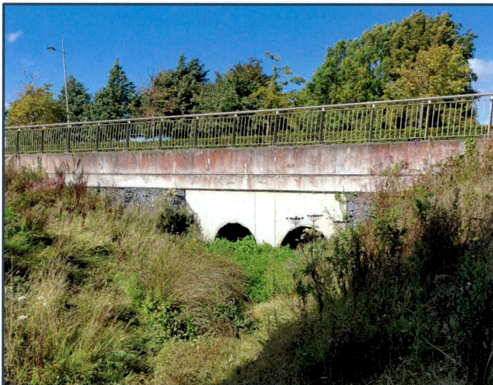
Figure 5-7 Upstream View of Culvert under Falcon Avenue
