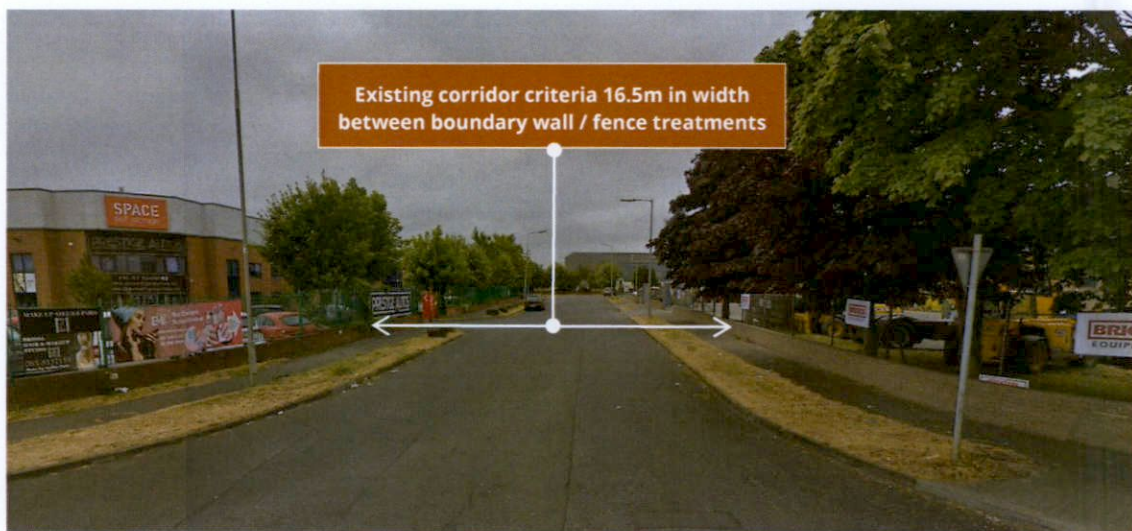
Figure 3.2: Existing Characteristics of Crosslands Business Park Access Road (Cul-De-Sac)
