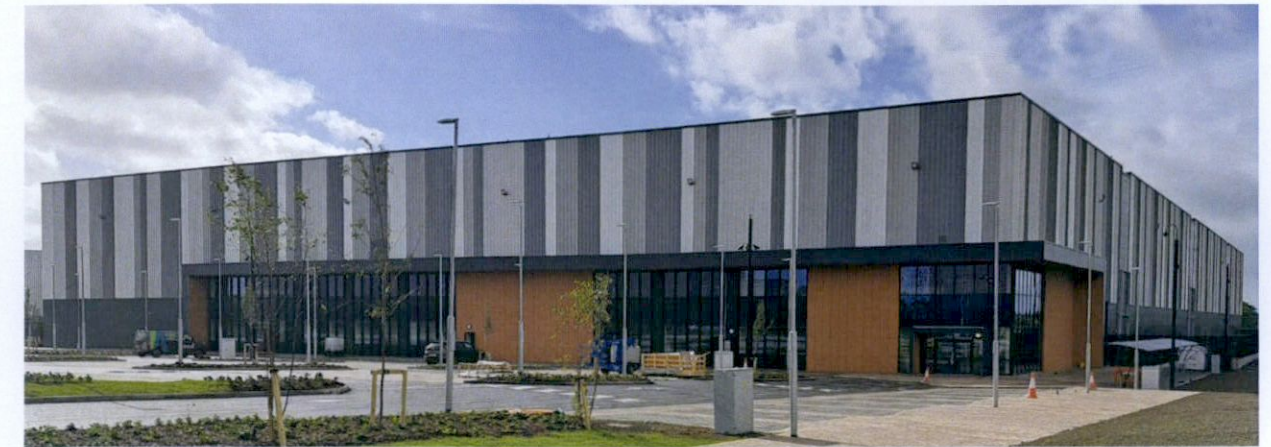
Photograph of logistic warehouse cladding precedent
