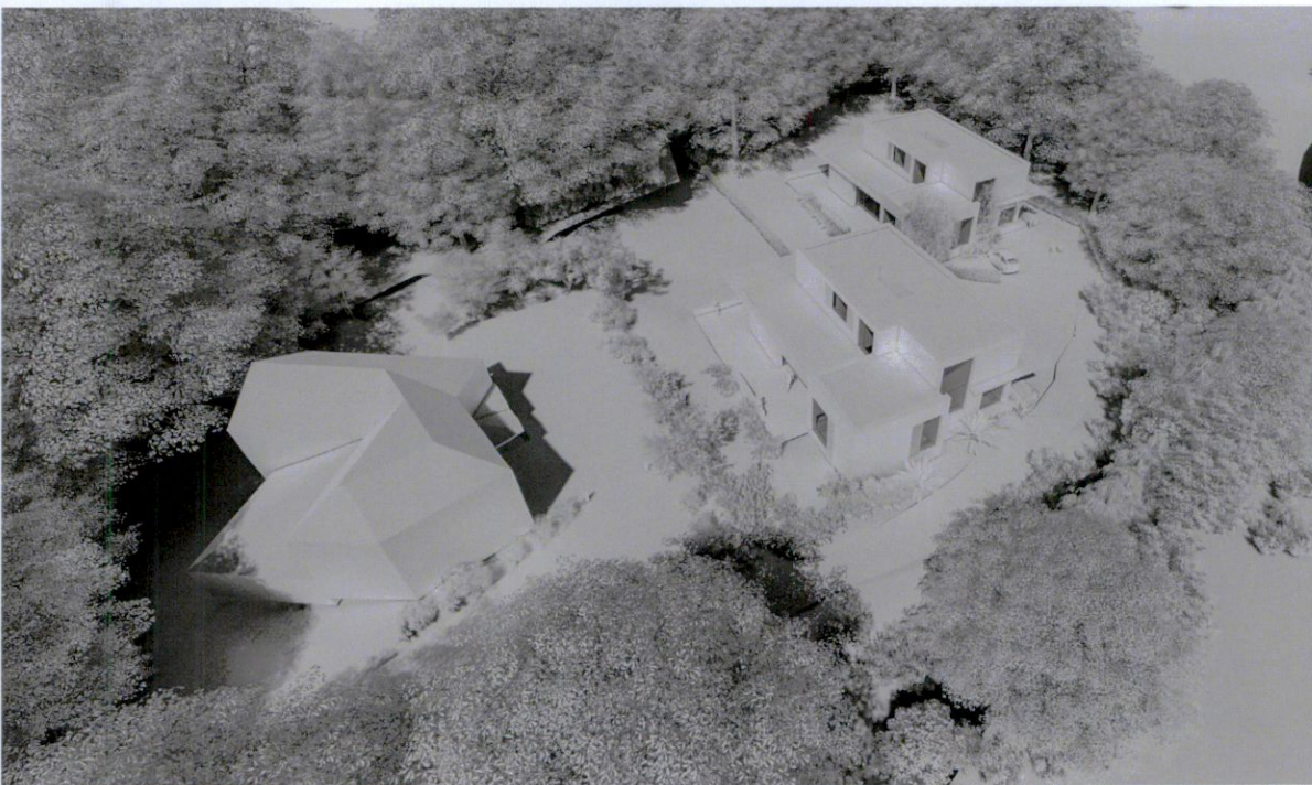
02 Aerial View of Proposal Looking North
