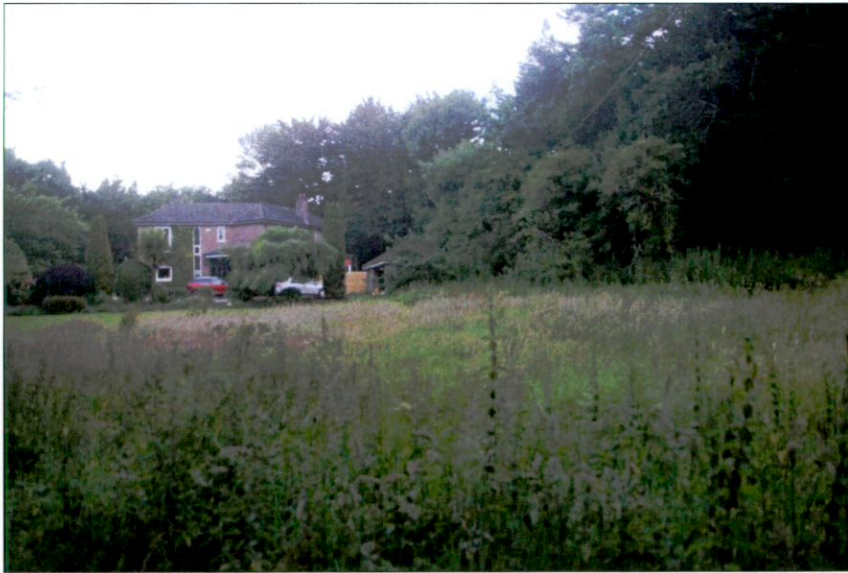
Plate 1 A view of existing building onsite (negligible bat roost potential, to be retained). Area to the front is the proposed footprint for development.
