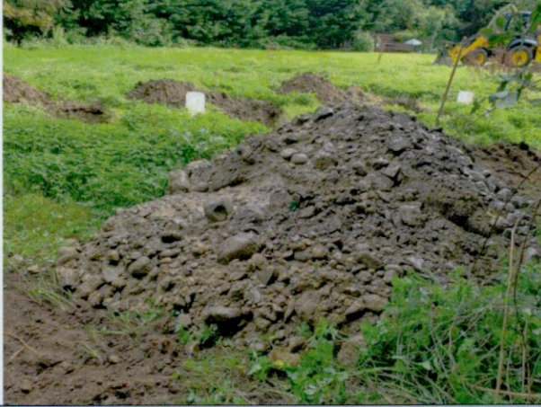
Trial Hole – Side View
