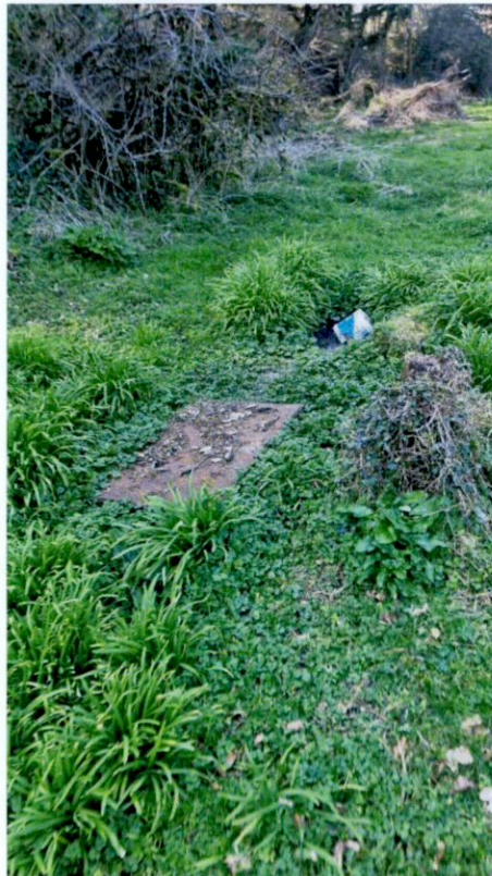
Existing Septic Tank to be Decommissioned
