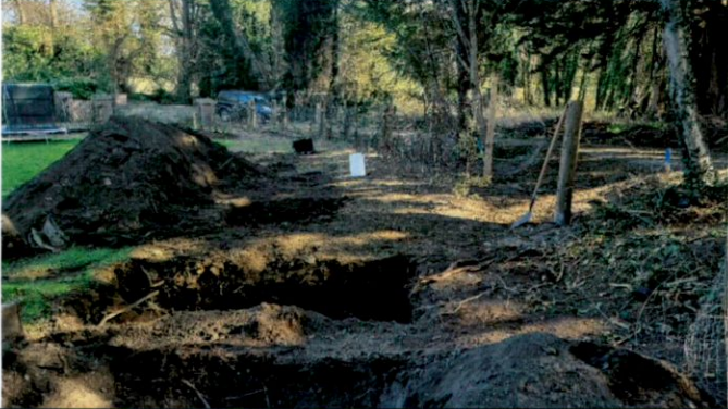
Trial Hole – Front View
