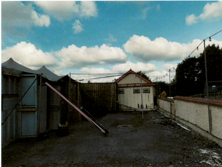
East Elevation of Temporary Toilets with Function Room beyond and Tent Structure to Side
