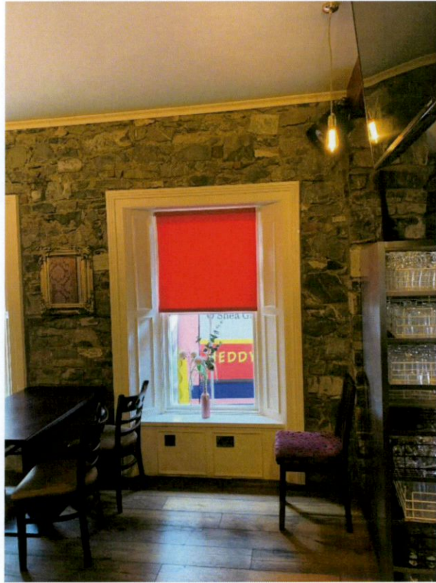
Internal View of Typical Window
