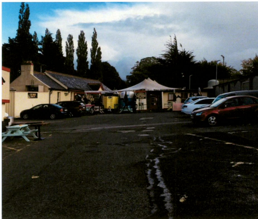
Part Elevation of Extension to Modern Extension to Salmon leap Inn in foreground with Function Room and Tent Structure beyond
