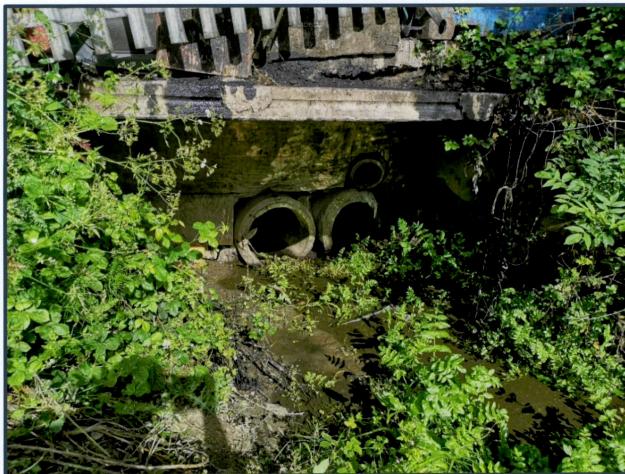
Figure 5-8 Inlet to twin-pipe culvert
