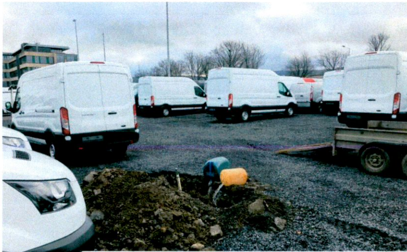
Site During Testing.
