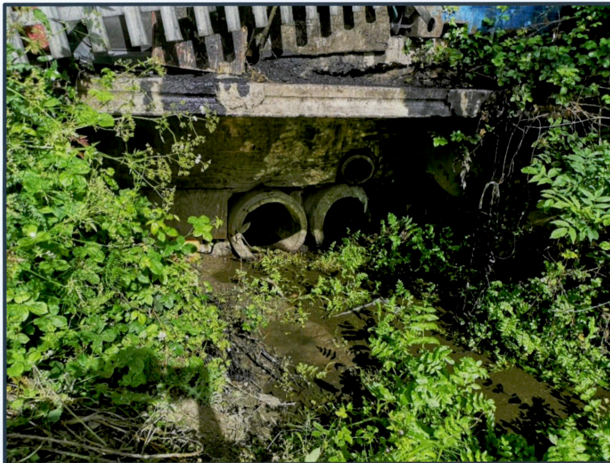
Figure 5-8 Inlet to twin-pipe culvert
