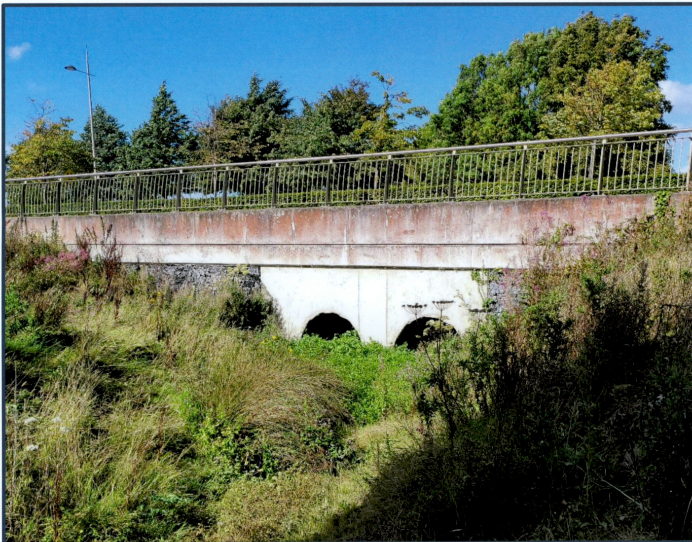
Figure 5-7 Upstream View of Culvert under Park Road
