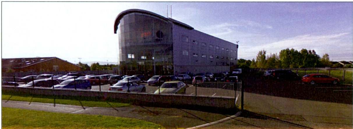
Figure 18.0 Image of constructed development c. 2009.
