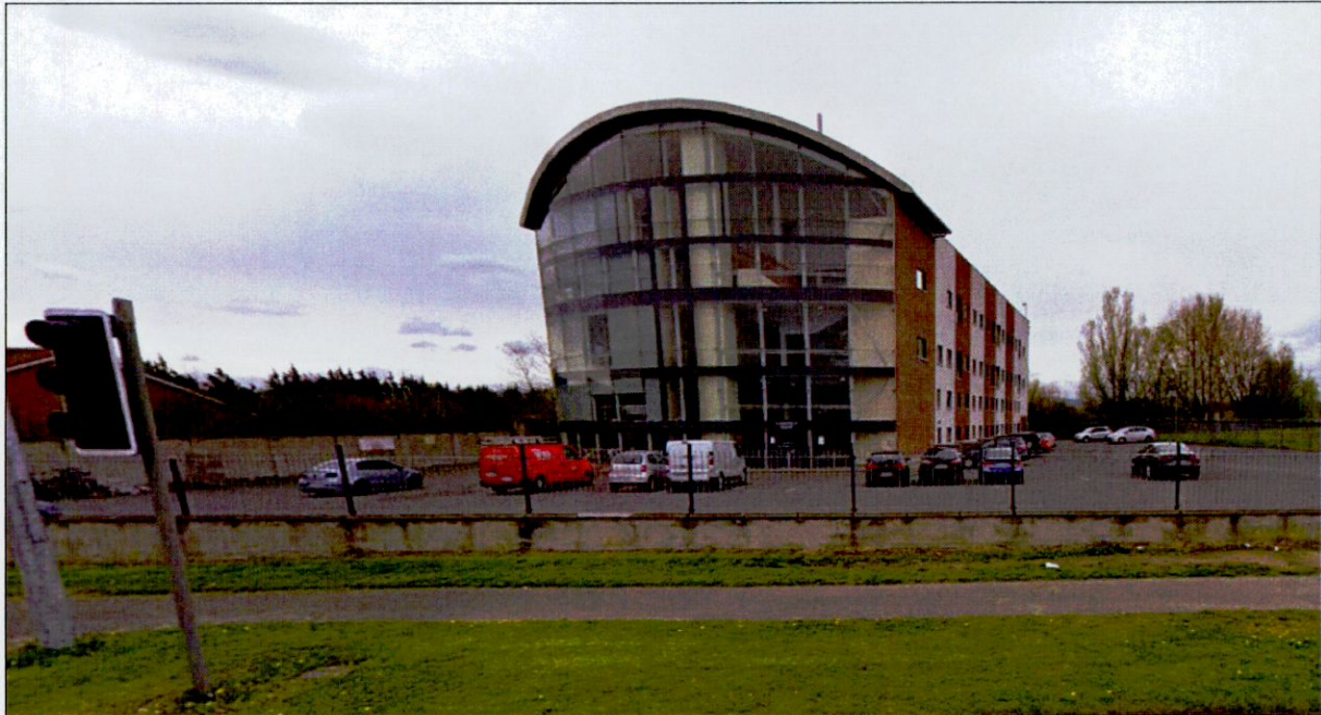
Figure 3.0 Street view image indicating the subject site (viewed from the north)
