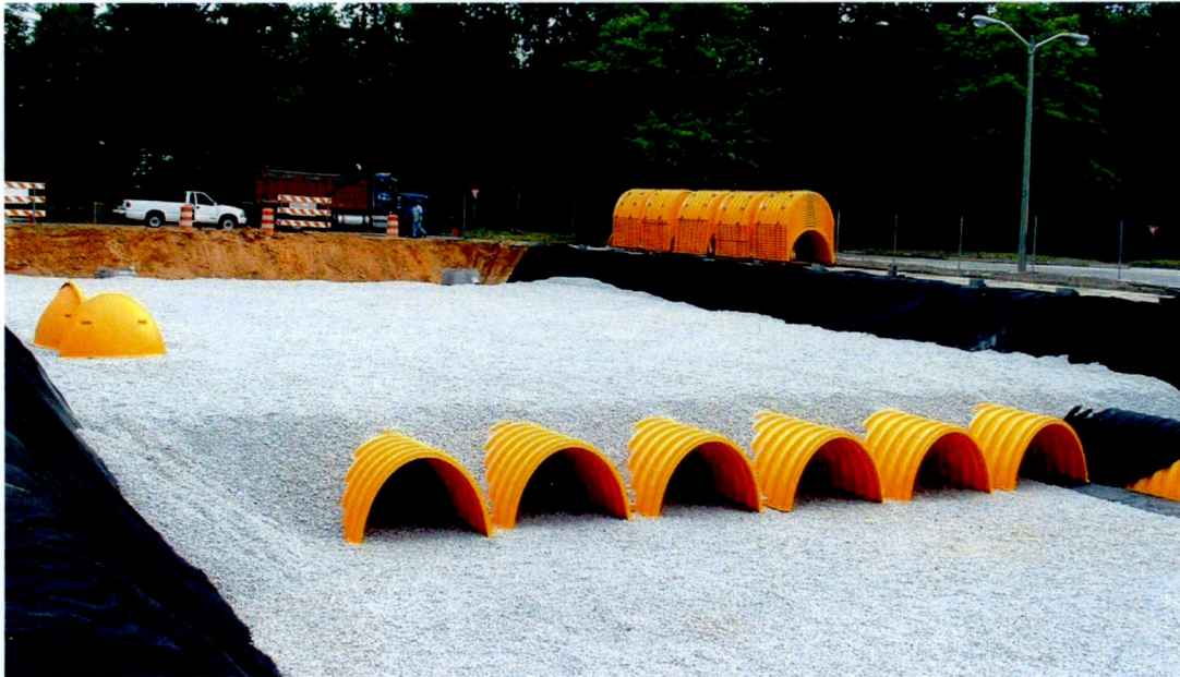
Figure 10 - Typical Cellular Storage (Stormtech) Installation
