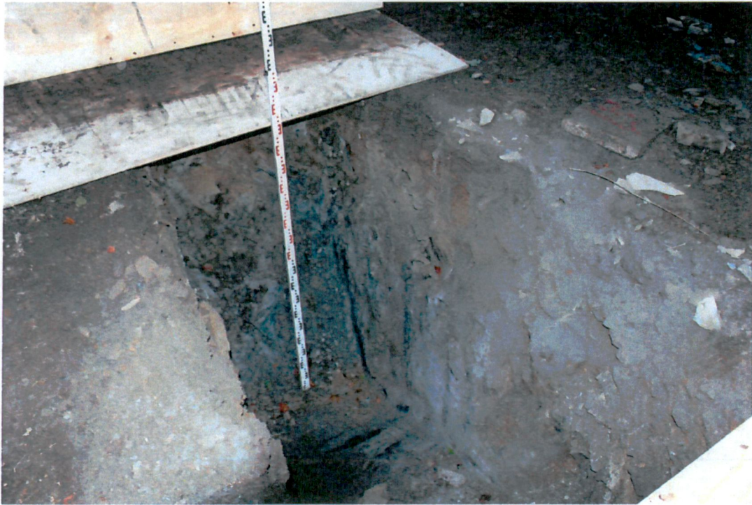
PHOTOGRAPH NO. 1 - TRIAL HOLE (300 mm Topsoil Removed)
