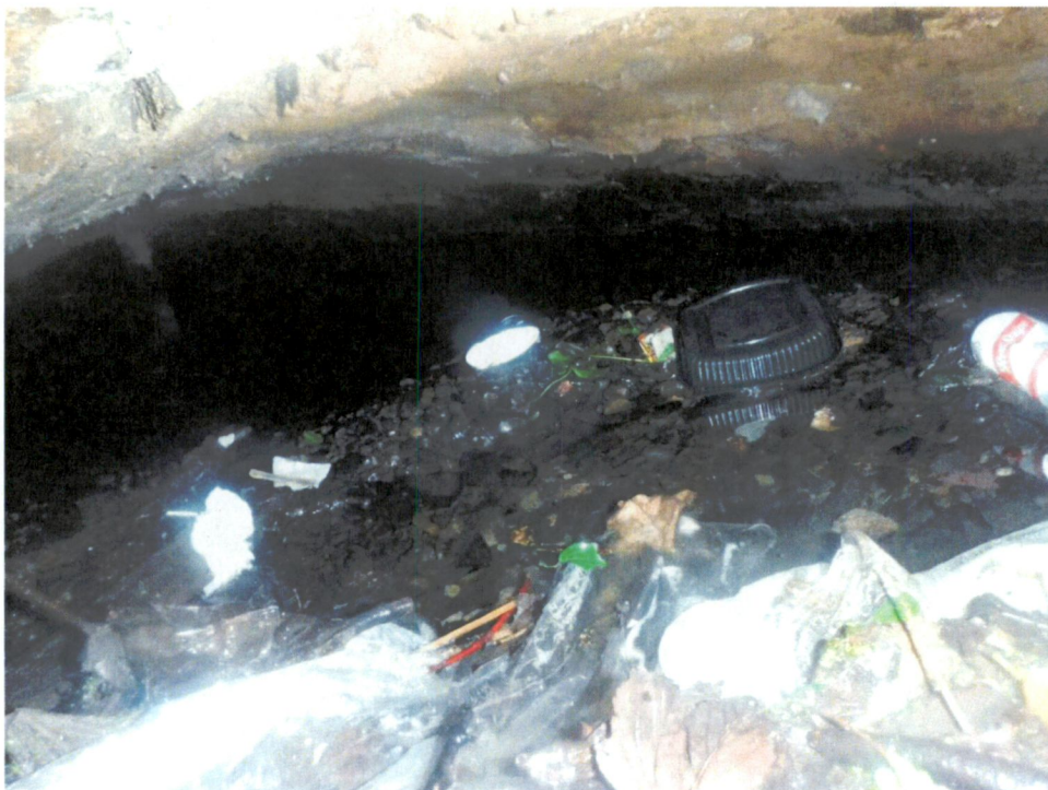
Photograph No. 4 Upstream End @ 2 m. Arch Barrel
