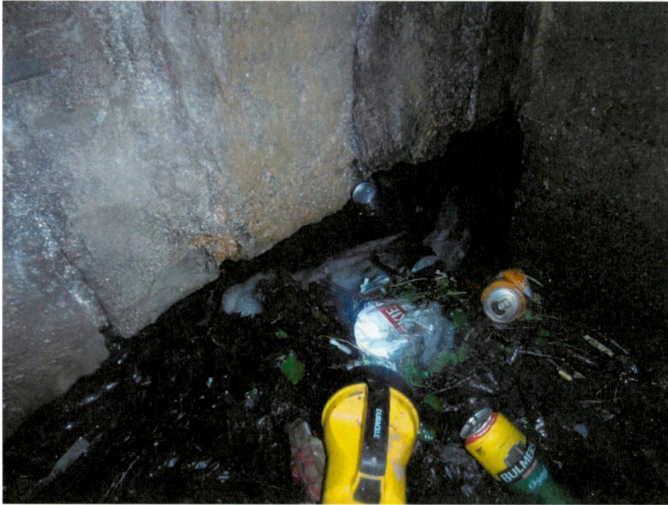
Photograph No. 1 Upstream end. Old bridge fascia.
