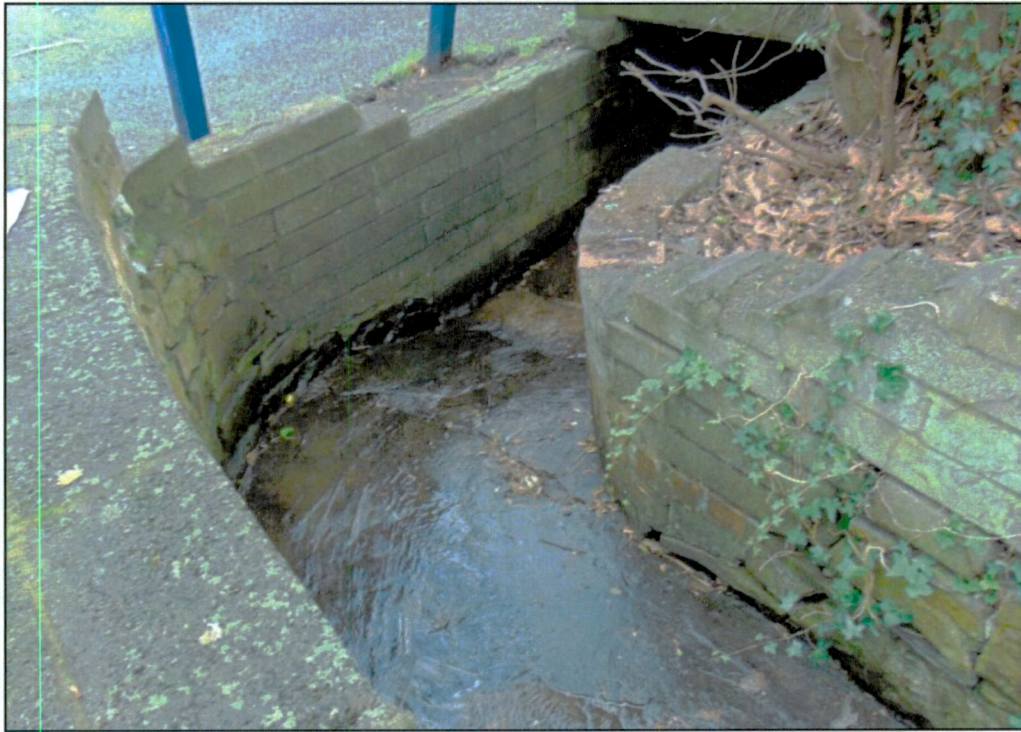
Photo 5: Stone Channel Downstream End
