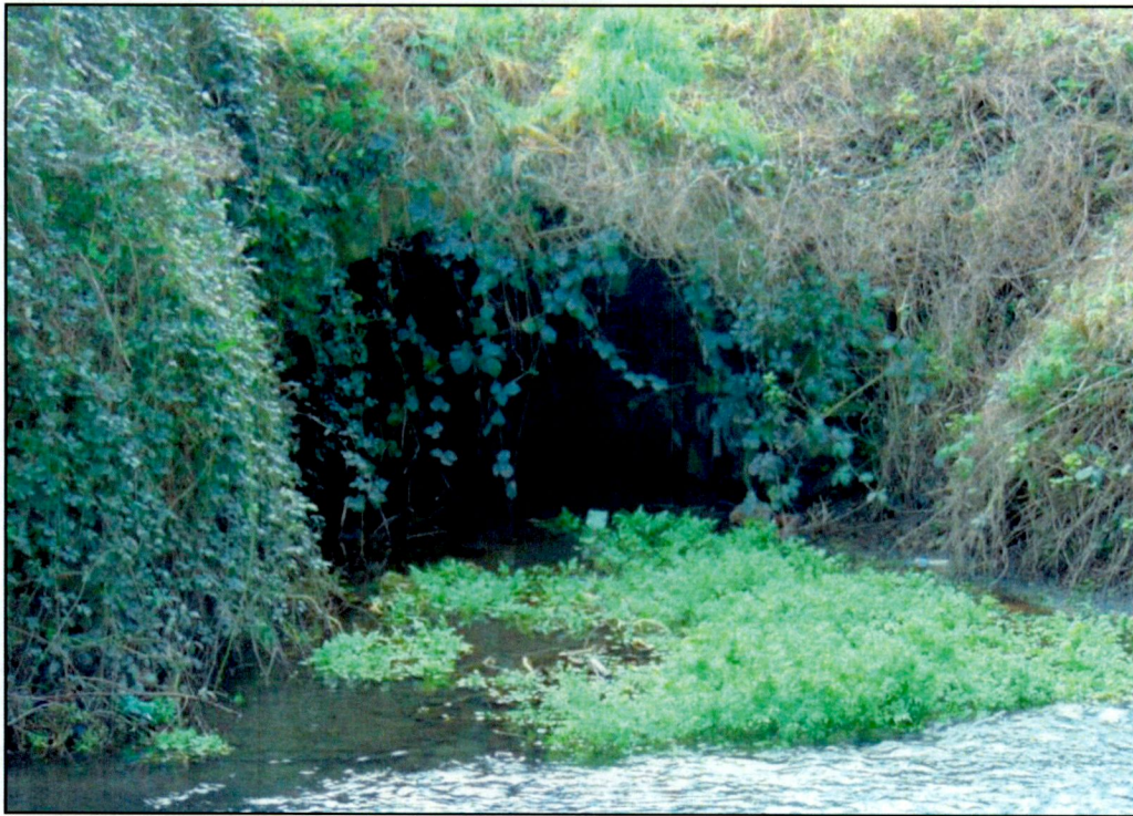
Photo 7: Culvert Outlet to Camac River
