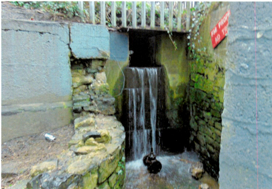
Figure 2 – Concrete Tank Outlet
