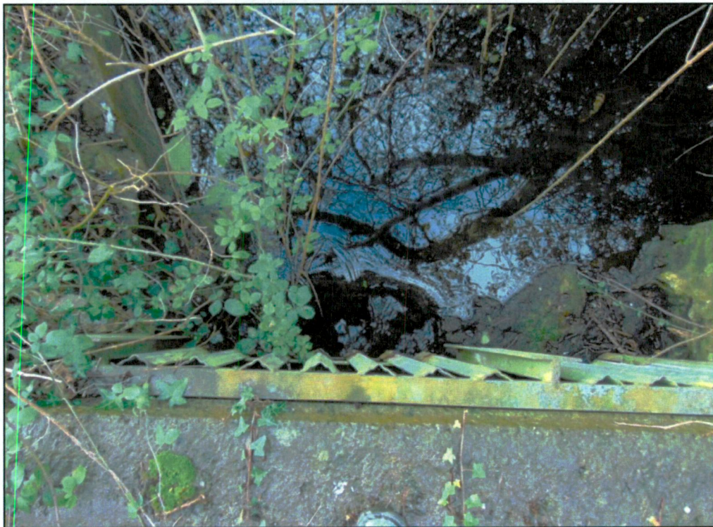
Photo 2: Pond Outlet into Concrete Tank
