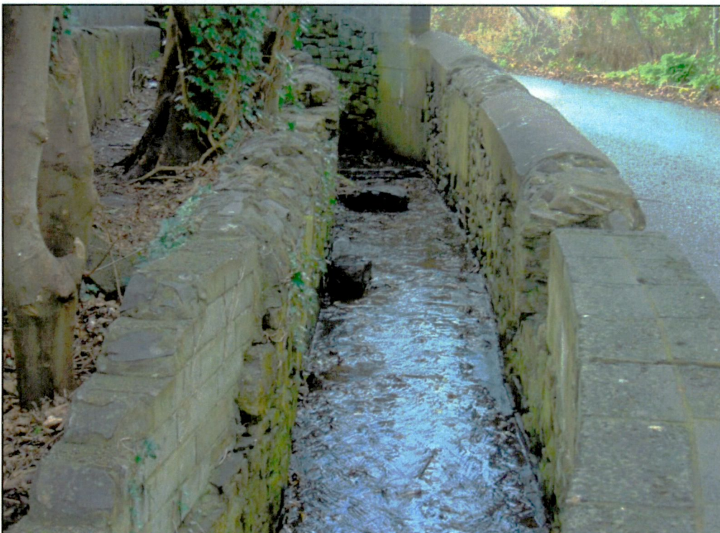
Photo 4: Stone Channel Upstream End
