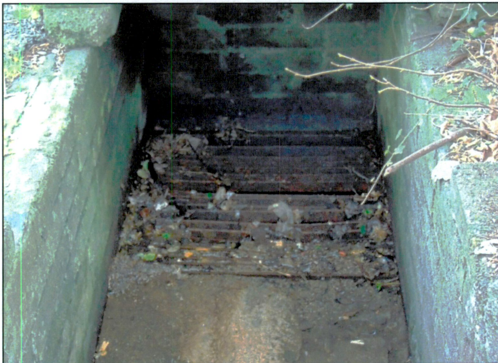
Photo 6: Sump Inlet & Grill
