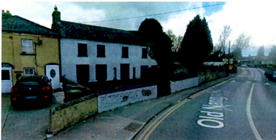
Unoccupied, boarded up House to East (RPS ref 136)
