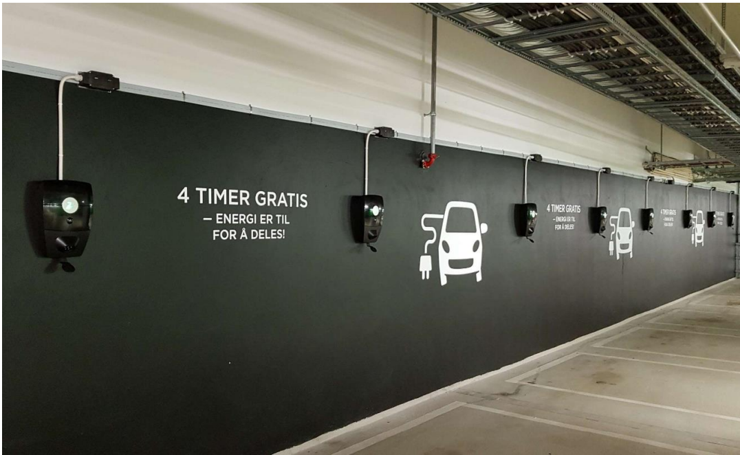
Figure 4 – Ziptec Pro Wall Mount Installation
