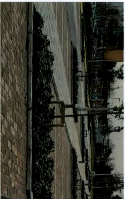
Permeable concrete paving to parking areas
