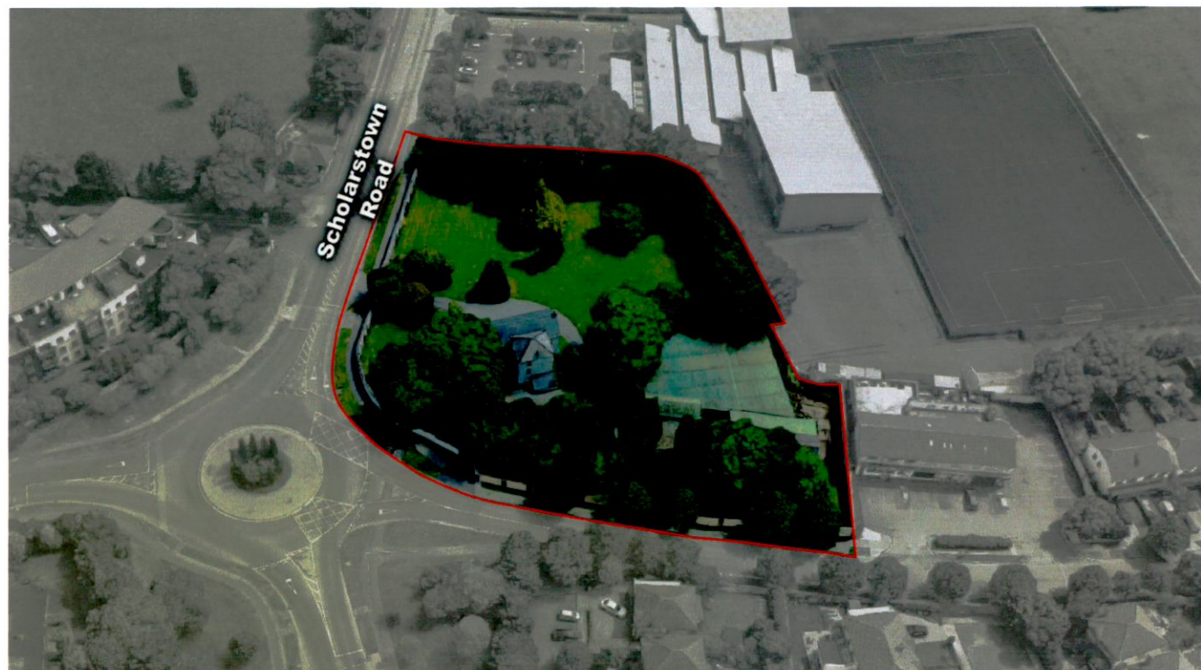
Aerial view from West of Site
