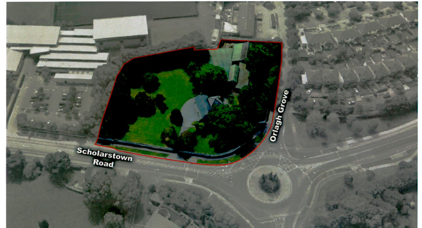
Aerial view from north of Site
