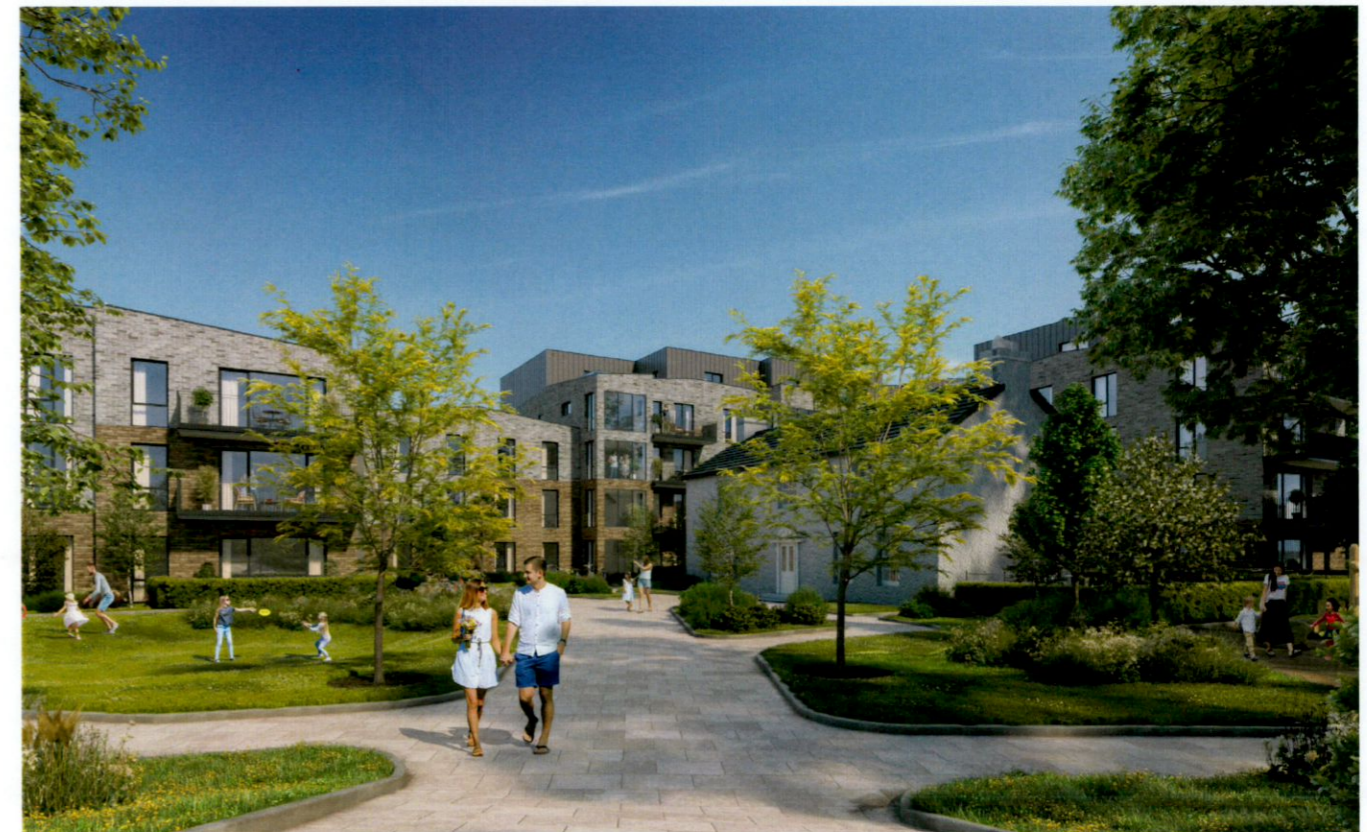
CGI View from North East: Scholarstown House with Contemporary New Build Backdrop
