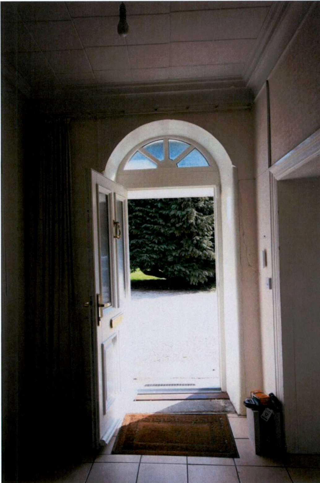
Plate 19: Entrance hallway looking to front door – note modern door and crude fanlight detail
