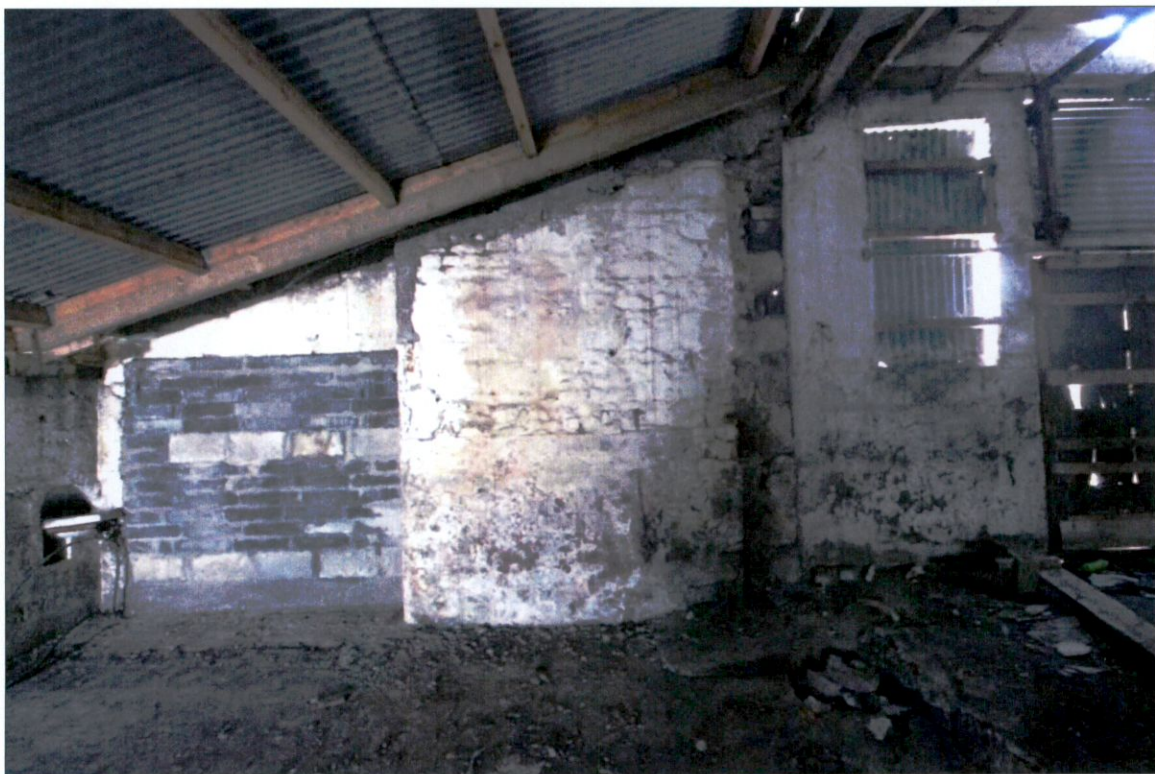
Plate 52: Interior of Building D1 looking south
