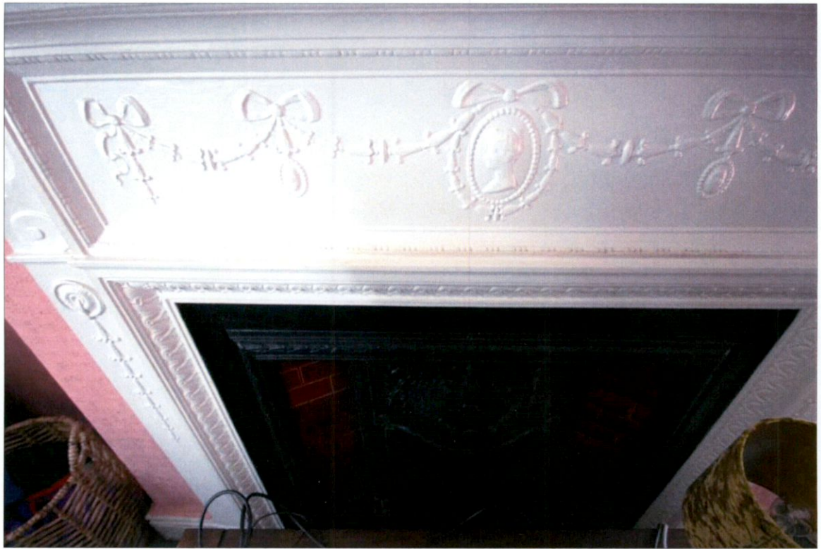
Plate 23: Edwardian fireplace detail in ground floor room GF02
