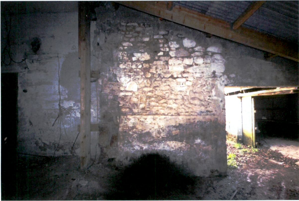
Plate 51: Interior of Building D1 looking north
