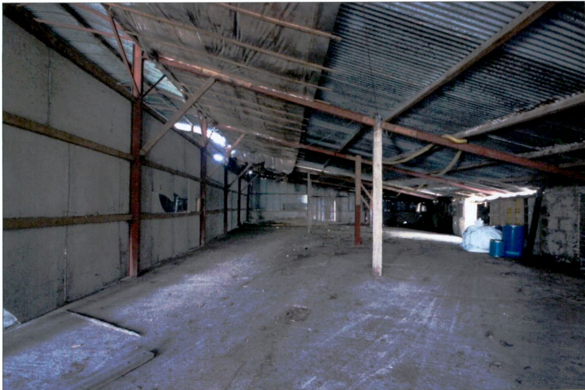
Plate 48: Interior of Building C
