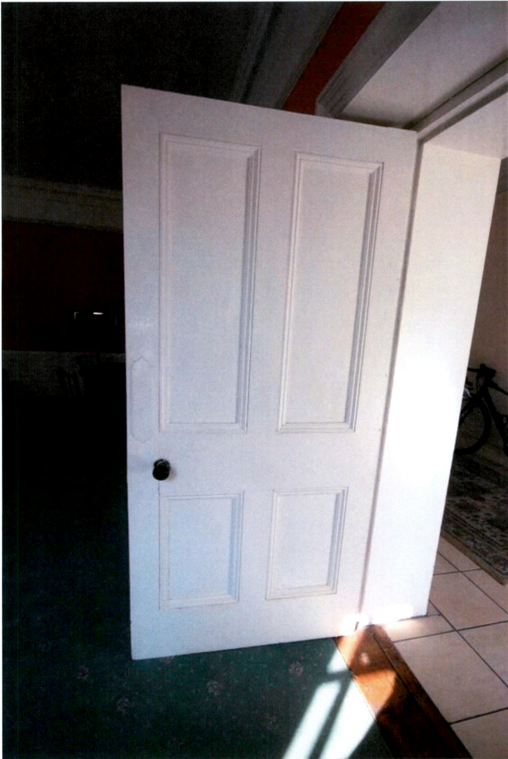
Plate 24: Painted timber four-panelled door in ground floor room GF02
