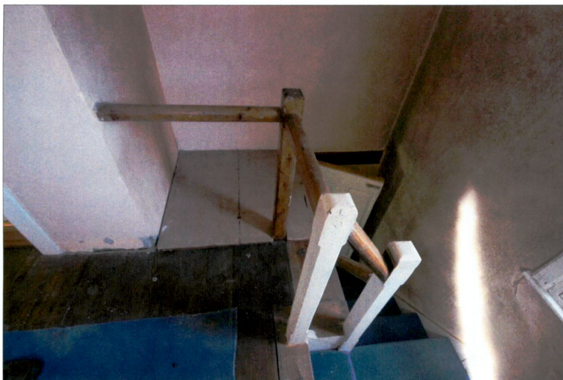
Plate 37: Staircase to second floor in return on landing SF01
