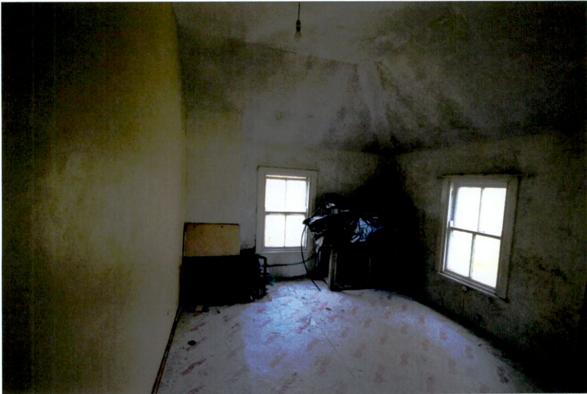
Plate 39: Second floor room in return SF03
