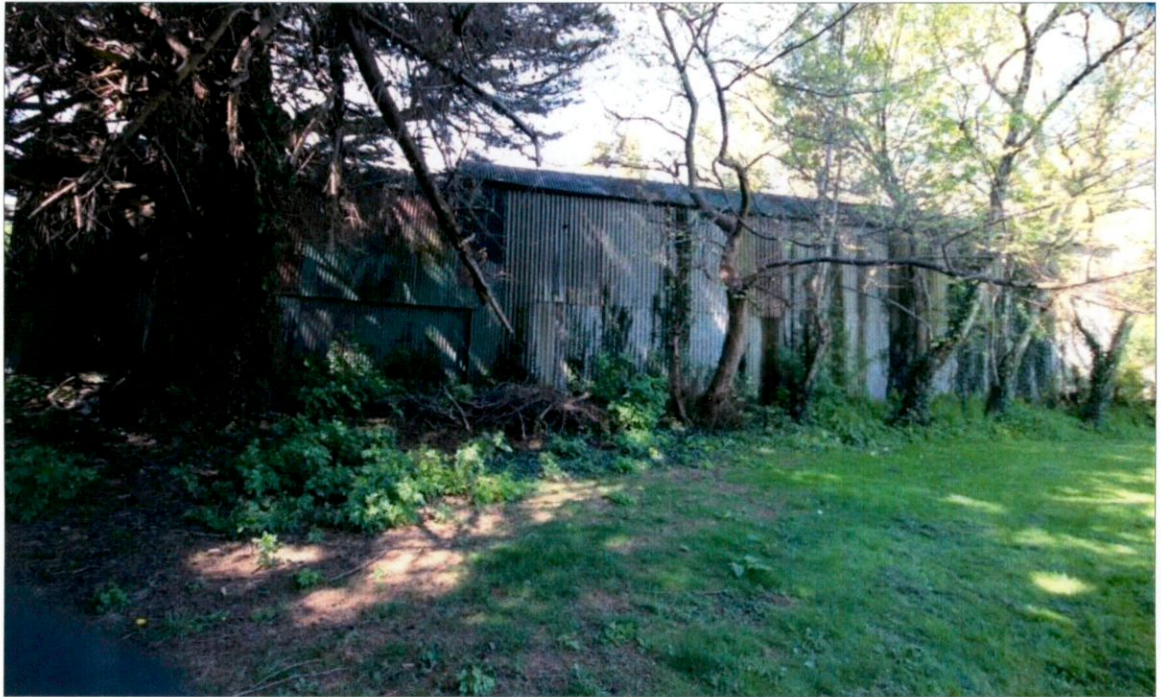
Plate 45: Eastern elevation of outbuildings
