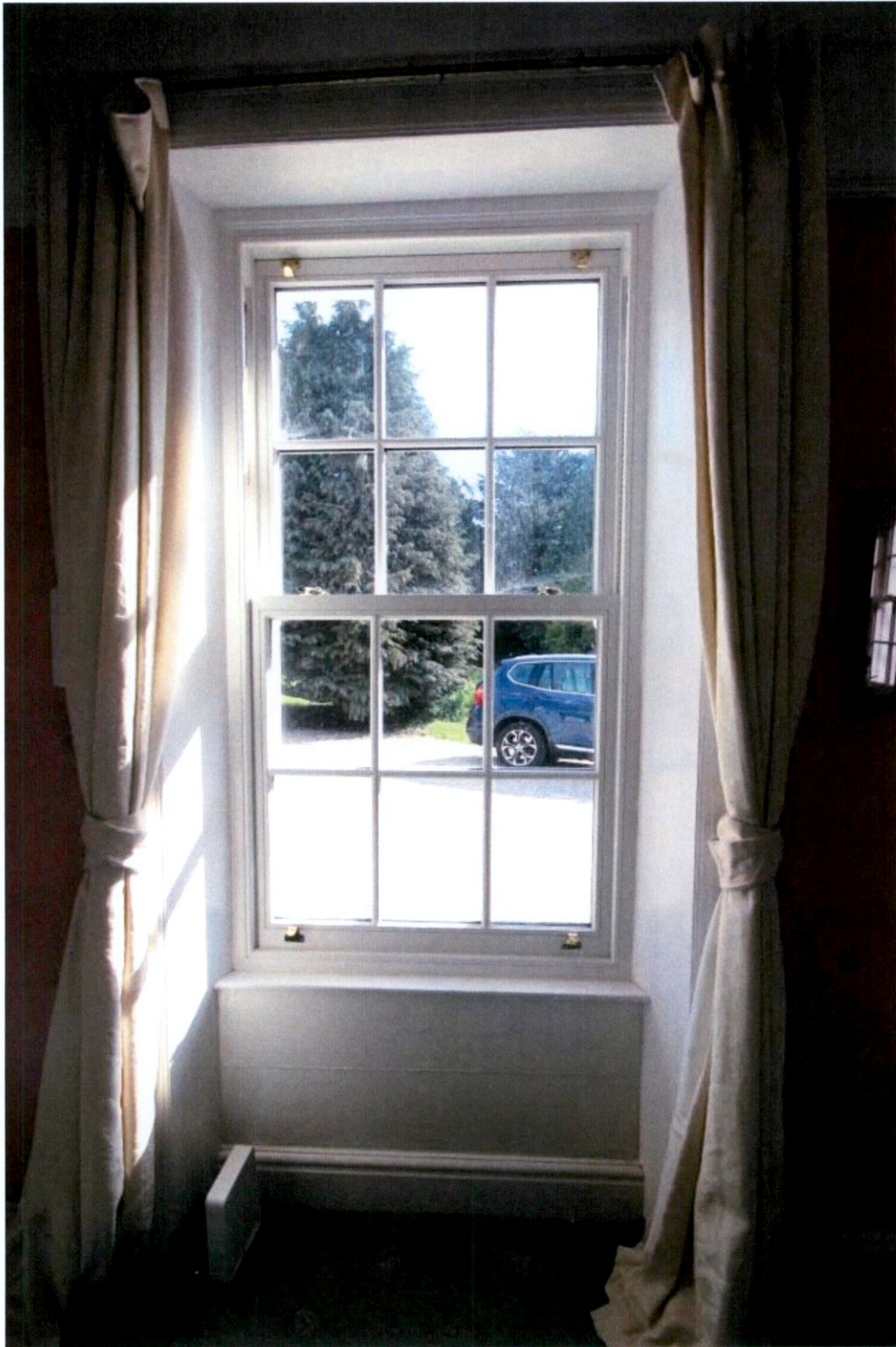
Plate 22: Typical replacement sash window to front elevation
