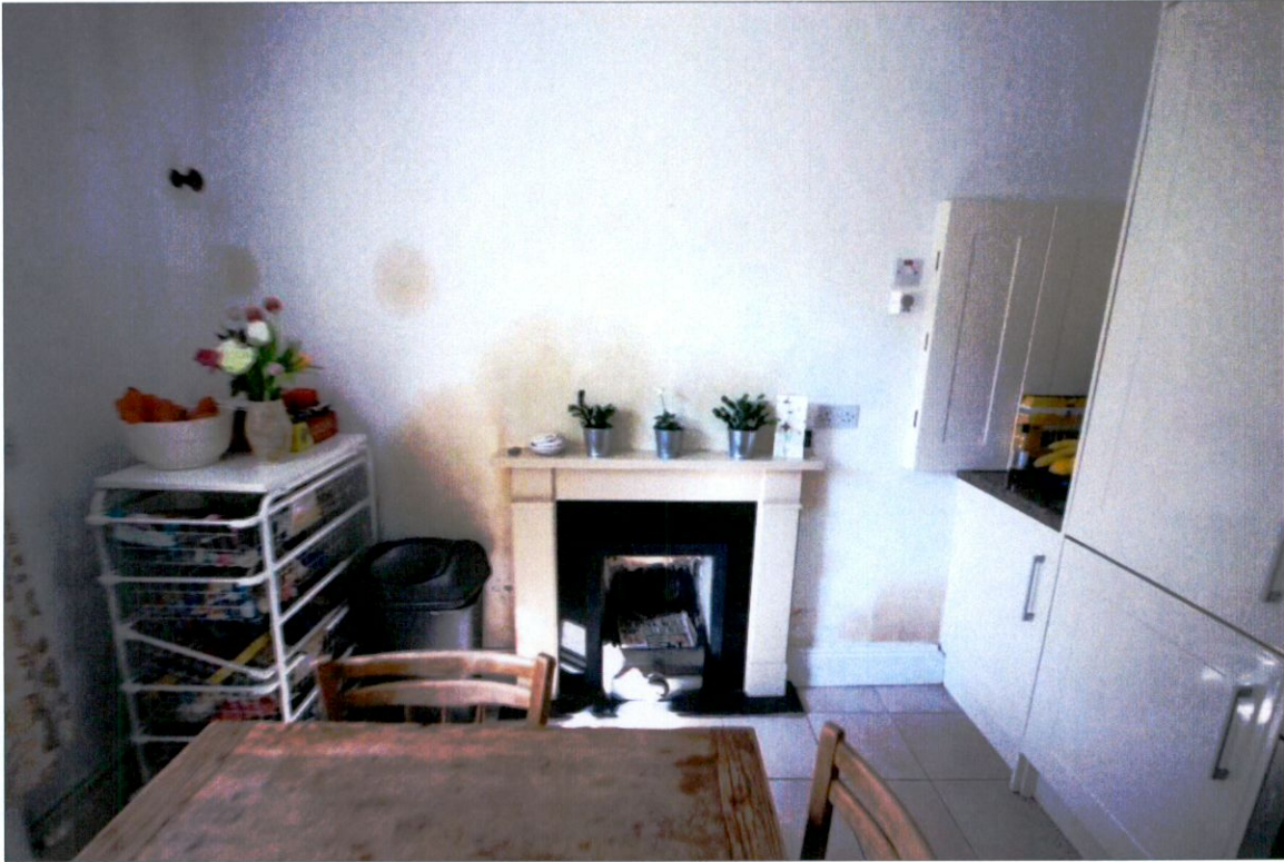
Plate 31: Kitchen in return GF05
