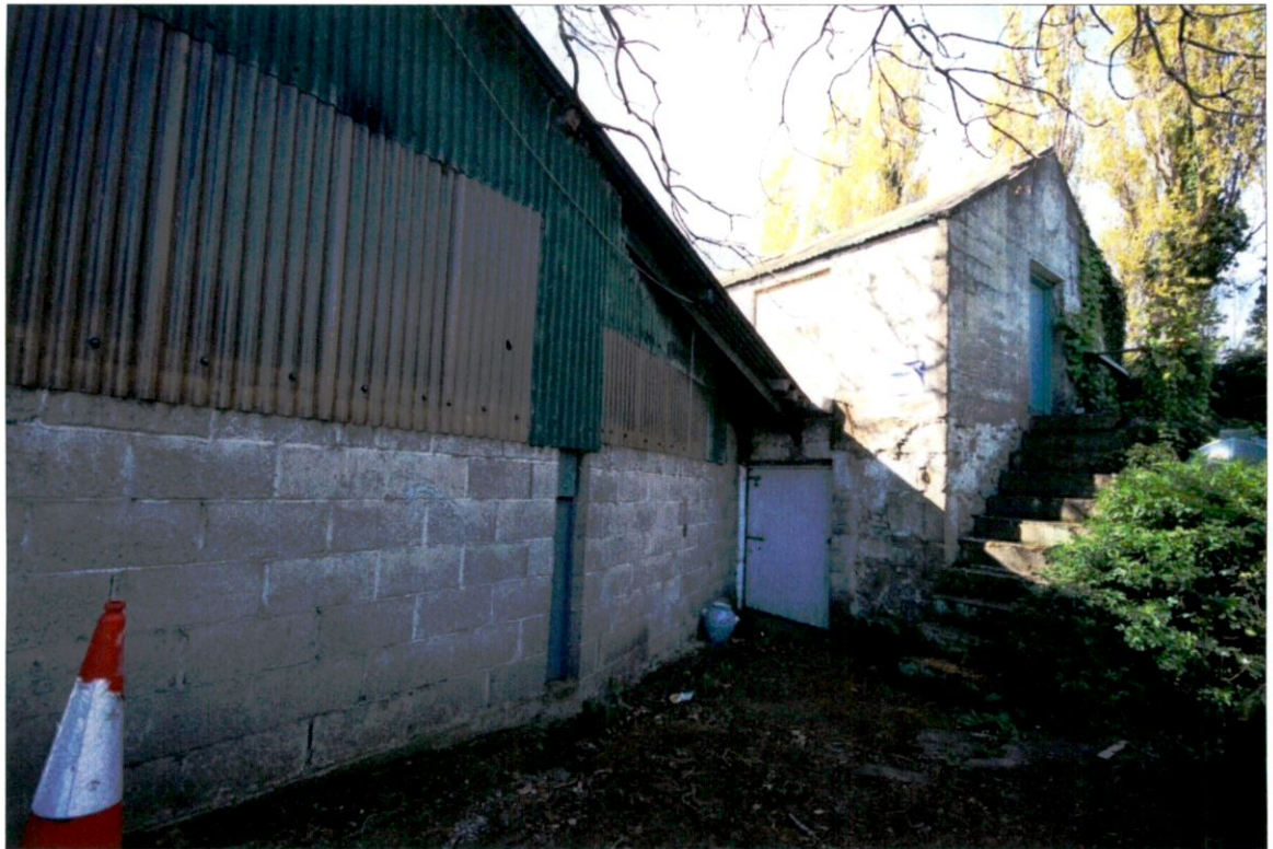
Plate 41: Northern elevations of outbuildings. Note rubble stone masonry walls to lower portion of building D2 with cast-concrete upper floor-level and steps.
