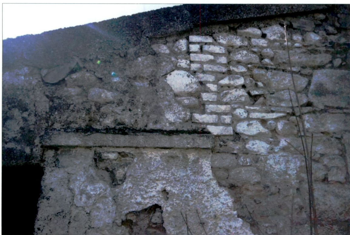
Plate 50: Northern elevation of Building D1 from internal yard
