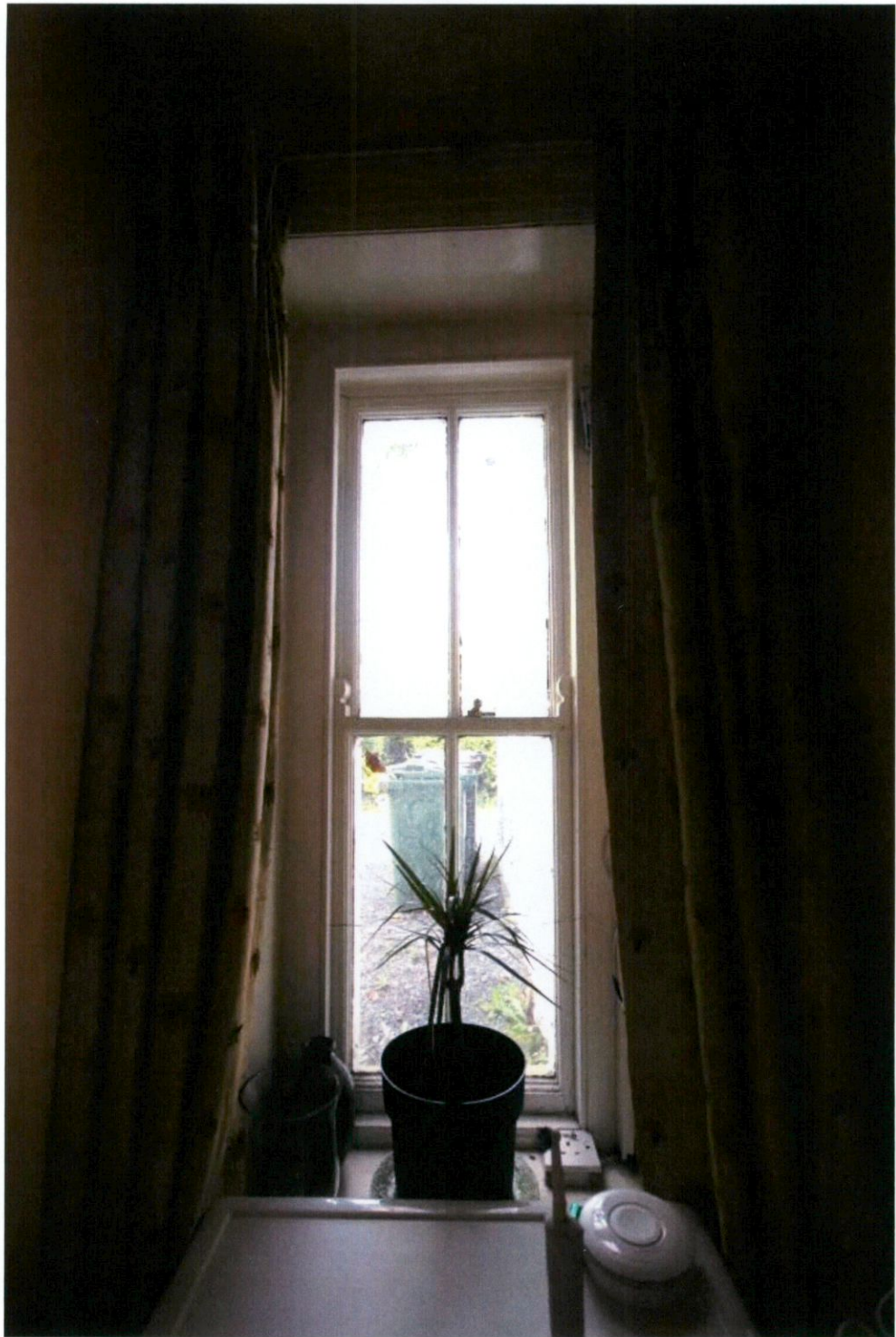
Plate 30: Painted timber sash window in GF04
