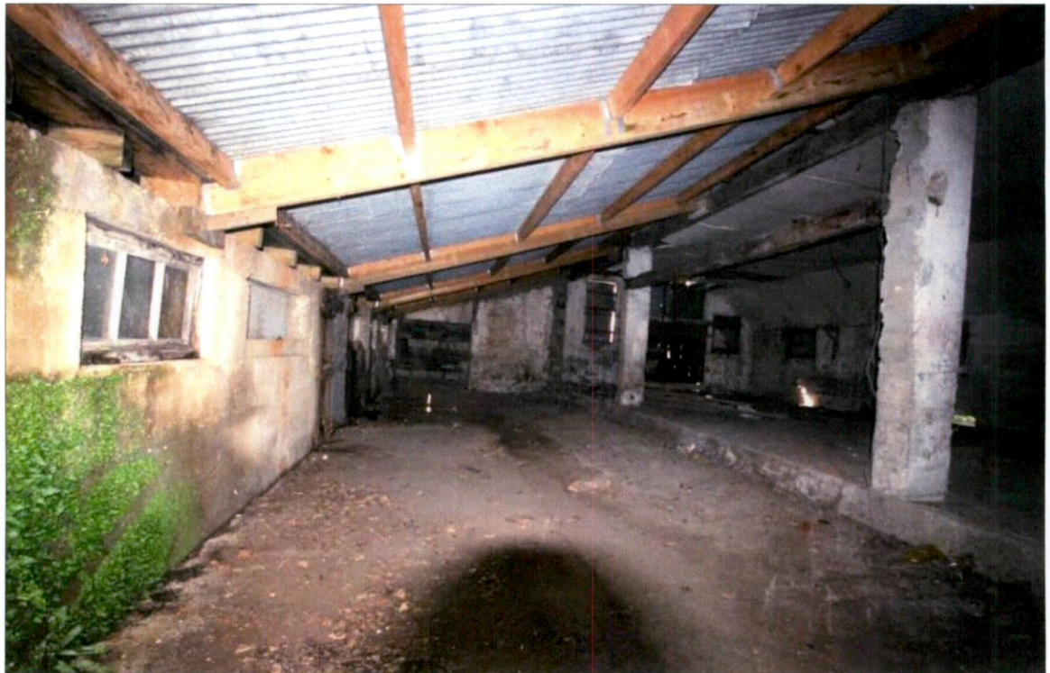
Plate 58: Interior of Building E southern end
