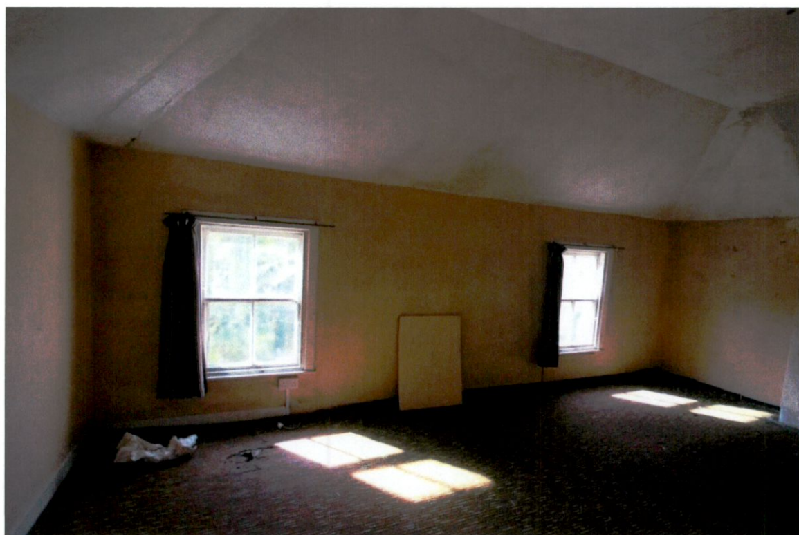
Plate 38: Second floor room in return SF02
