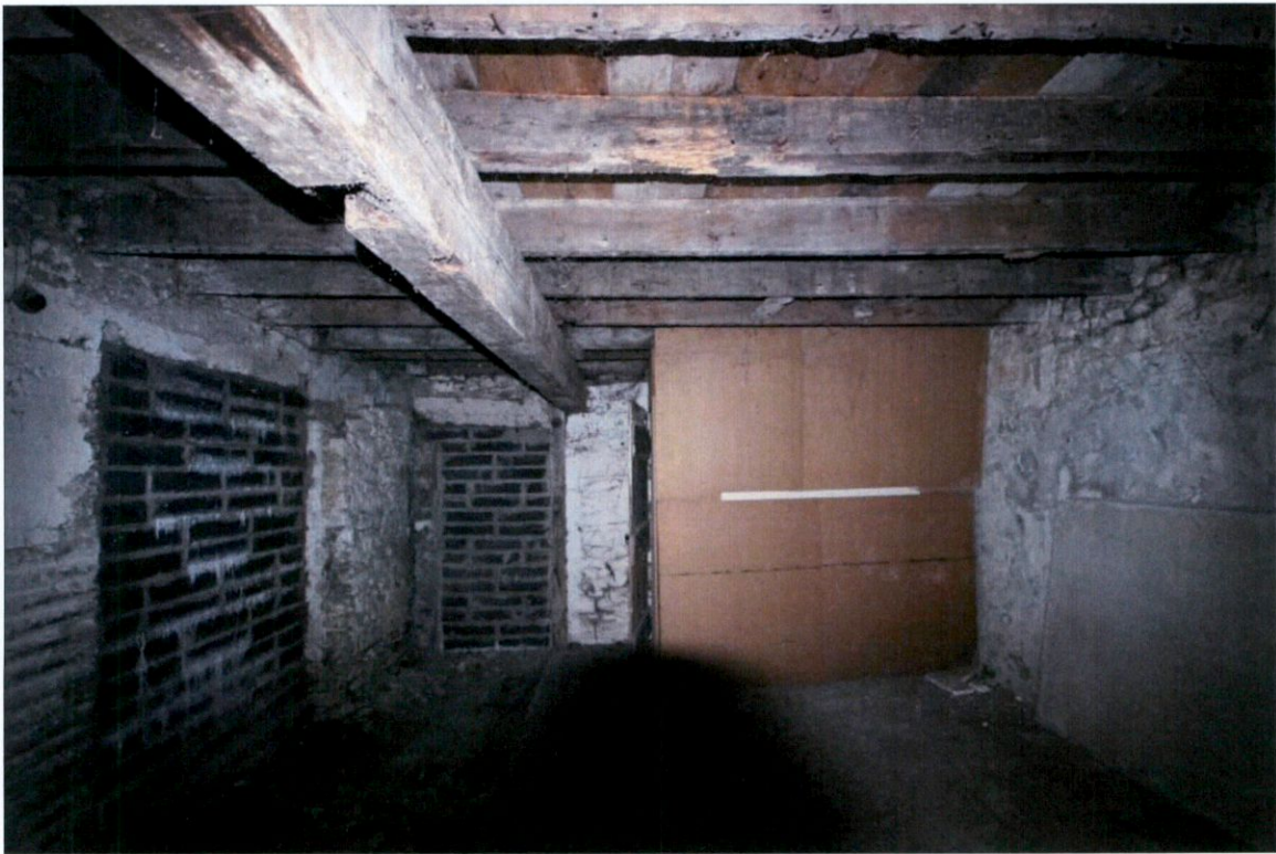
Plate 54: Interior of Building D2 looking south
