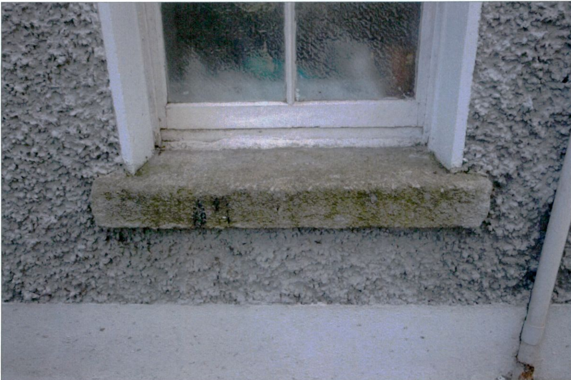
Plate 17: Granite sill to ground floor window to rear return
