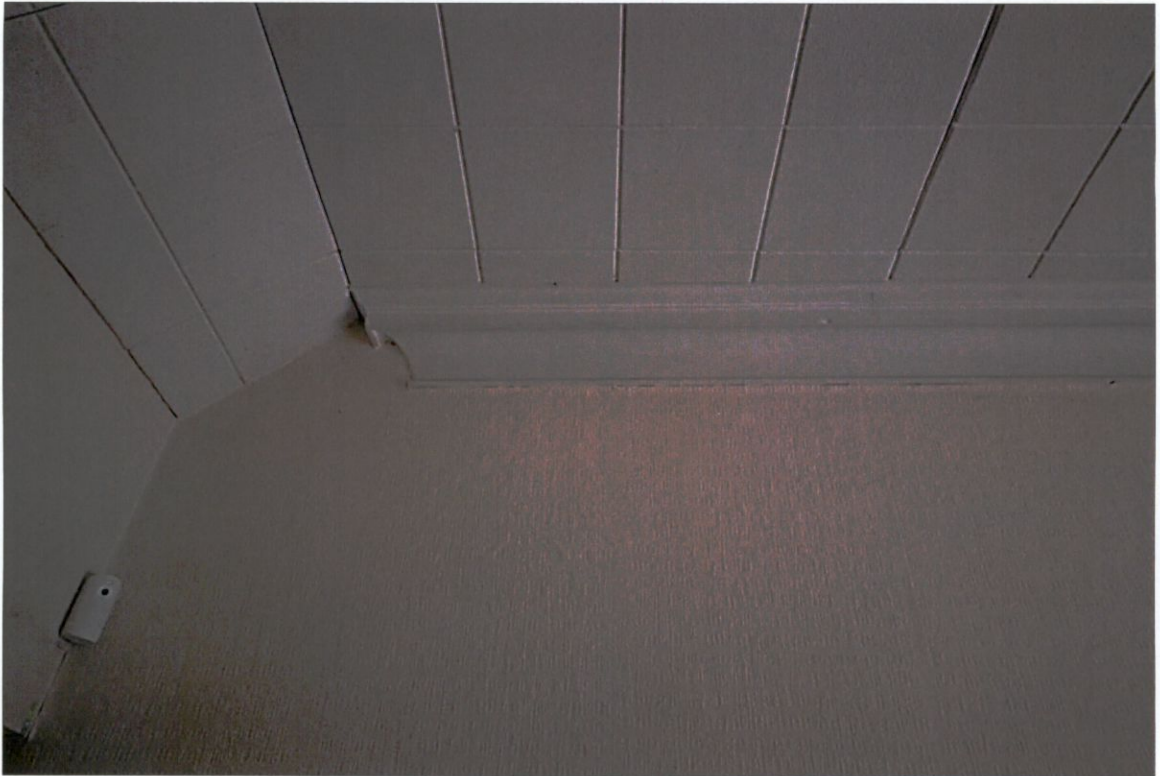
Plate 20: Cornice detail in entrance hallway GF01
