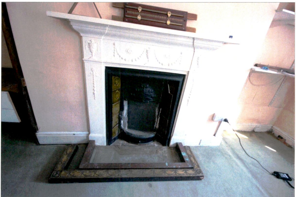
Plate 26: Fireplace in ground floor room GF03
