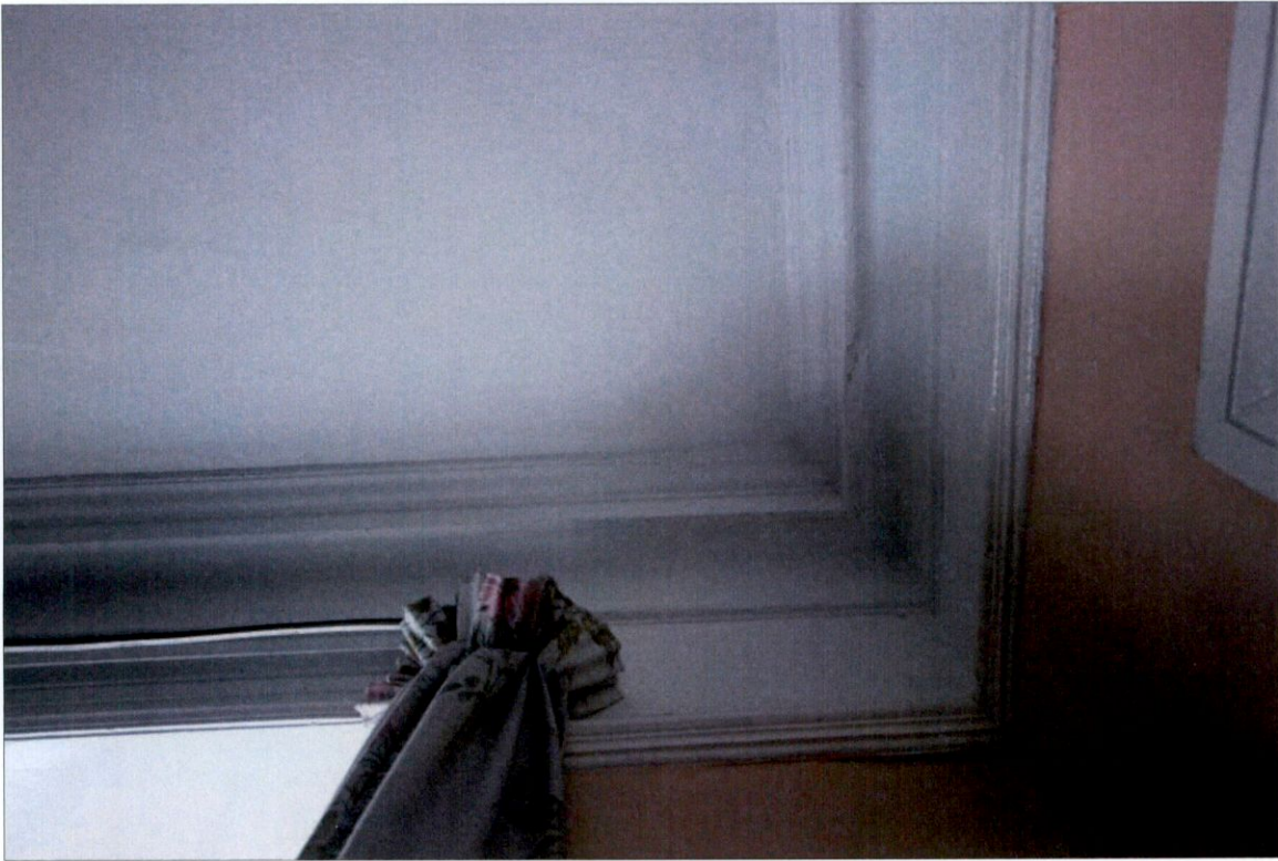
Plate 27: Cornice detail in ground floor room GF03
