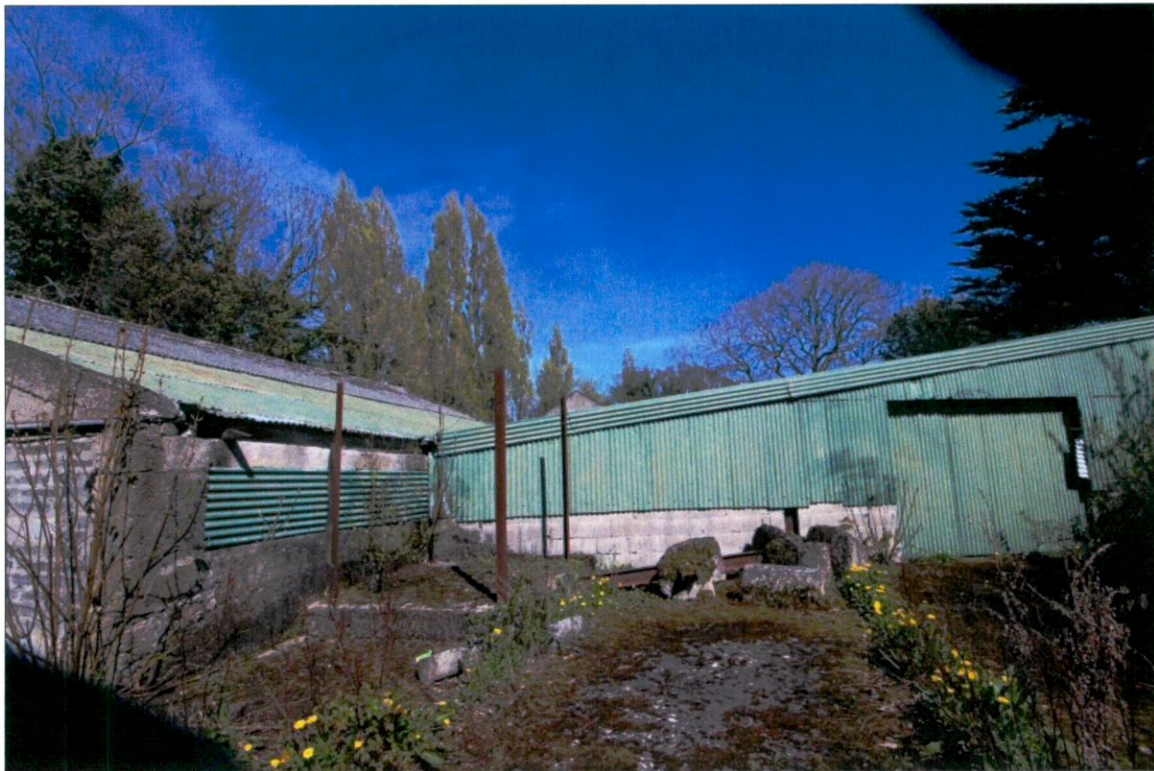
Plate 44: Southern elevation of outbuildings
