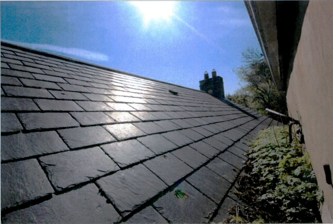
Plate 16: Valley between main roof and return
