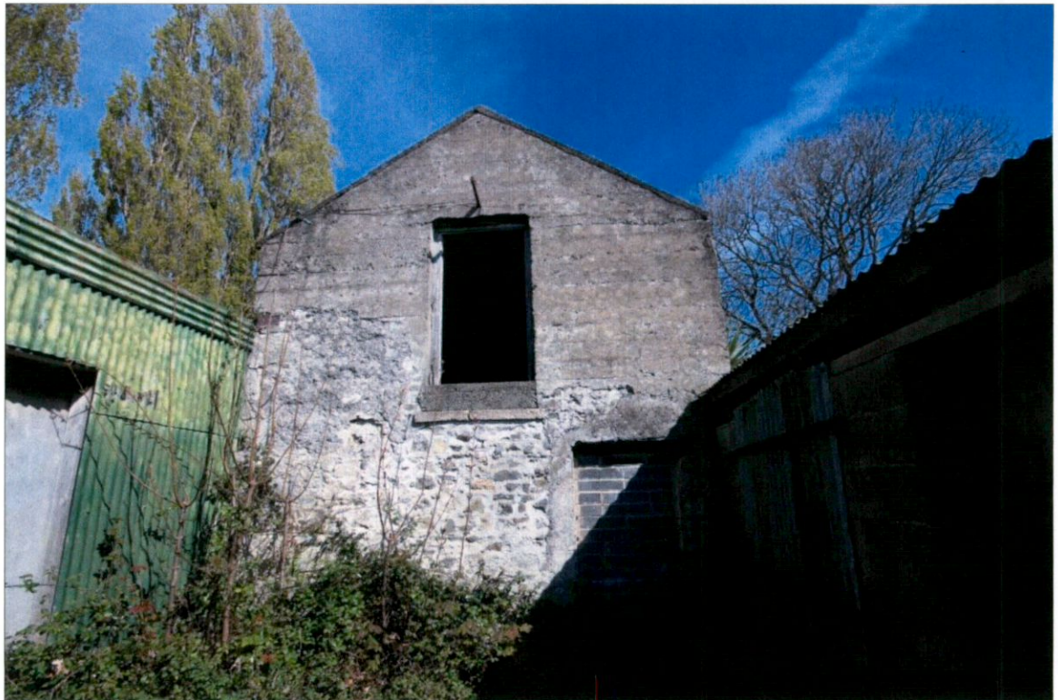
Plate 46: Southern elevation of two-storey building D2 from internal open yard
