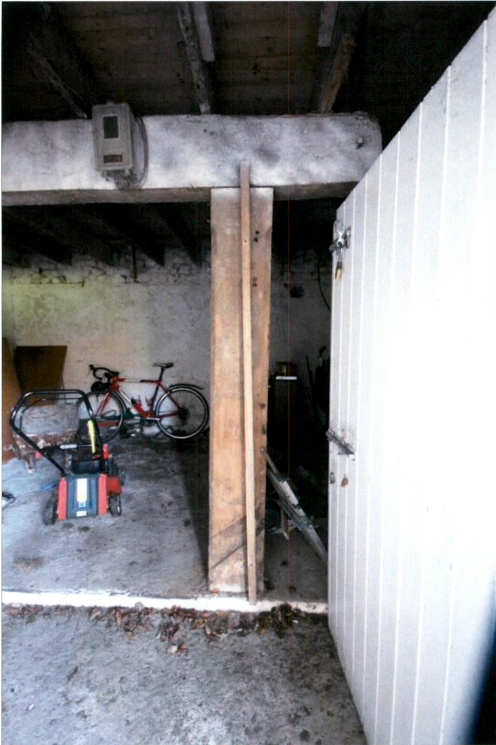
Plate 55: Oak beams in Building D2
