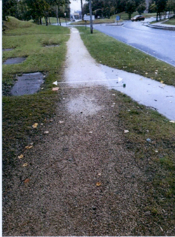
Figure 11: Widen 0.3m to RHS. Chainage ~ 180.0m. Arrowed line 2m wide.
