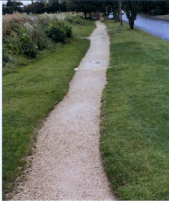
Figure 3: Widen 0.8m to RHS. Chainage ~ 40.0m. Arrowed line 2m wide.
