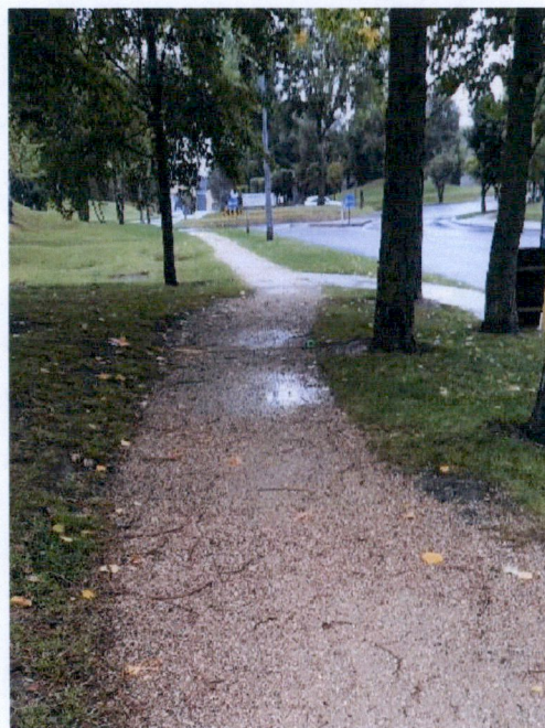
Figure 9: Widen 0.3m to RHS and LHS. Chainage ~ 160.0m. Arrowed line 2m wide.
