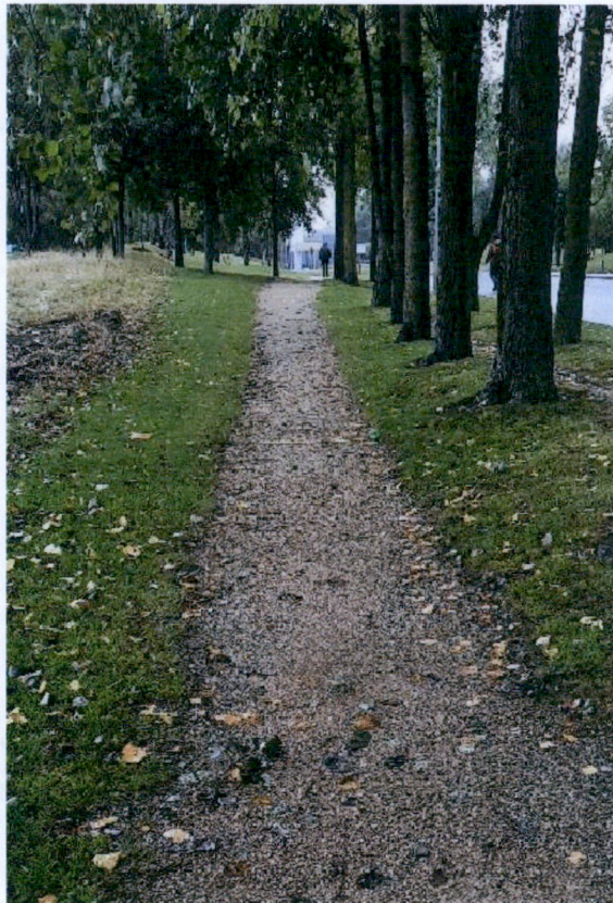
Figure 8: Widen 0.8m to LHS to avoid roots. Chainage ~ 140.0m. Arrowed line 2m wide.
