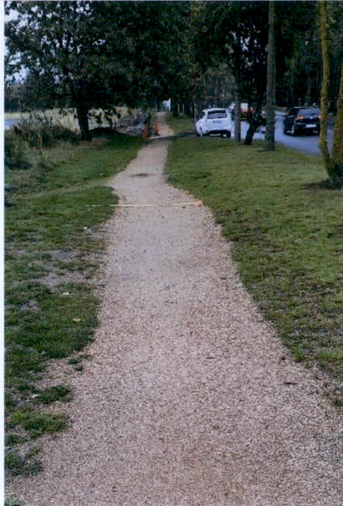
Figure 5: Widen 0.3m to LHS to limit impact on roots. Chainage ~ 60.0m. Arrowed line 2m wide.
