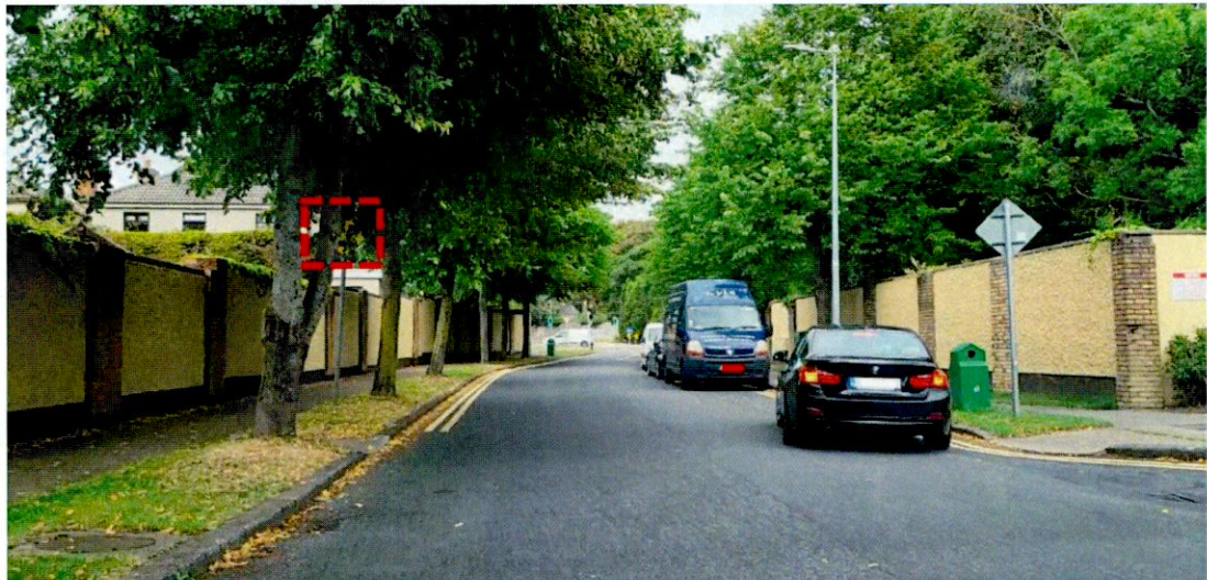
Figure 22: Existing Warning Sign for roundabout ahead is Obstructed
