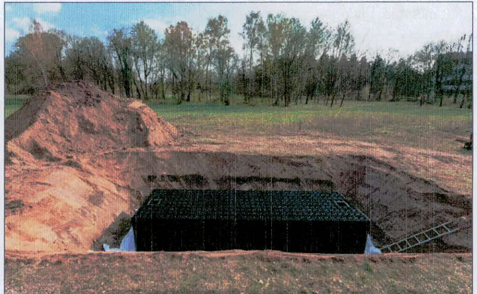
Stormbloc® Optimum installation.
