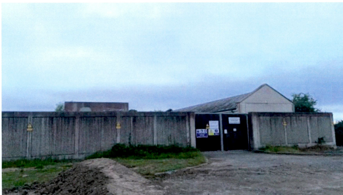
The substation where Leisler's bat activity was very much in evidence
