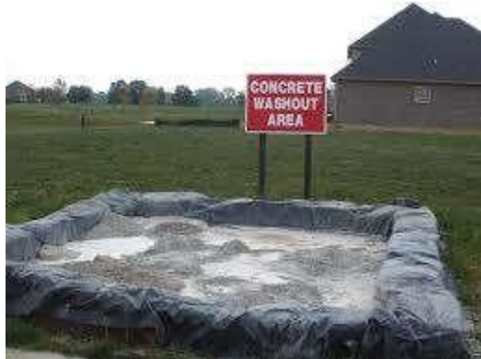
Figure 5-4 Example of temporary concrete washout area
